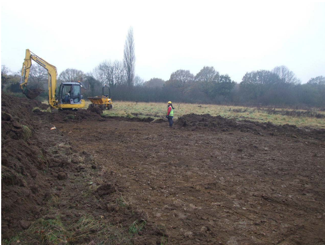
Fig 2 Thames Water compound, Ockham, looking west
