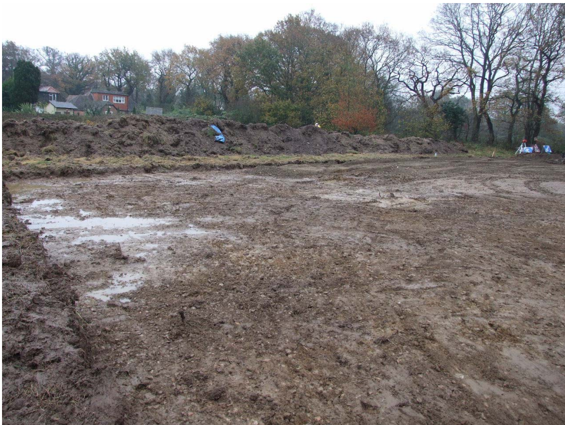
Fig 3 Thames Water compound, Ockham, looking east
