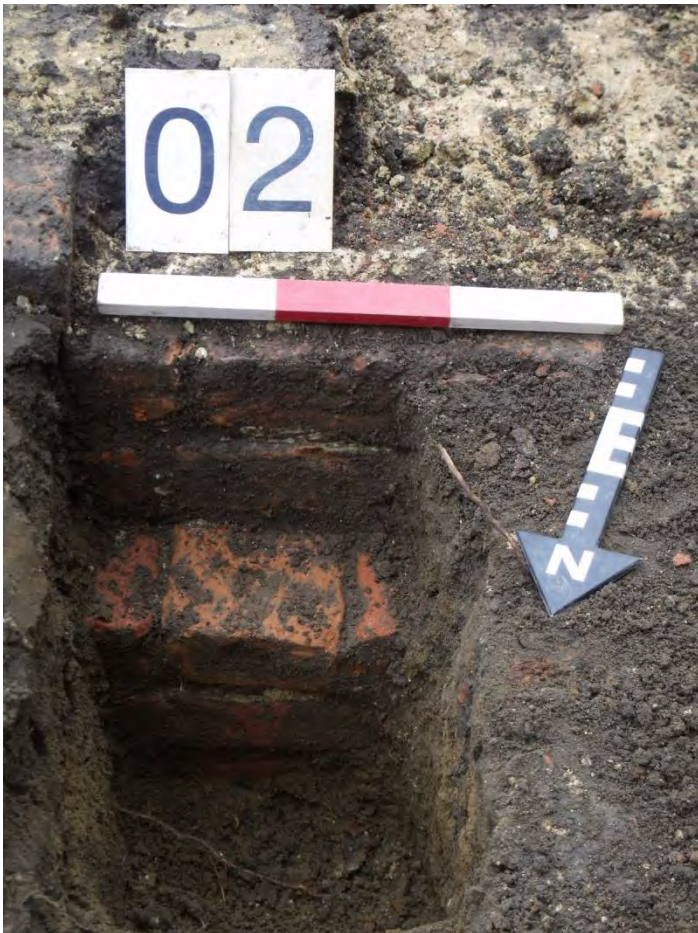
Fig 9 Reigate Priory Junior School, Reigate; Stepped foundation, wall <02>. View to the south.
