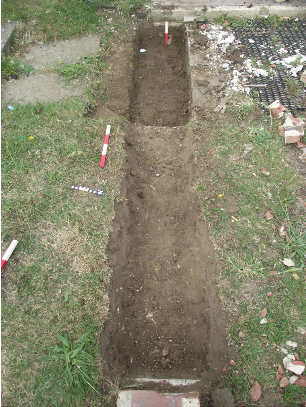
Fig 5. Shepperton Primary School, Shepperton. Strip foundation 1.
