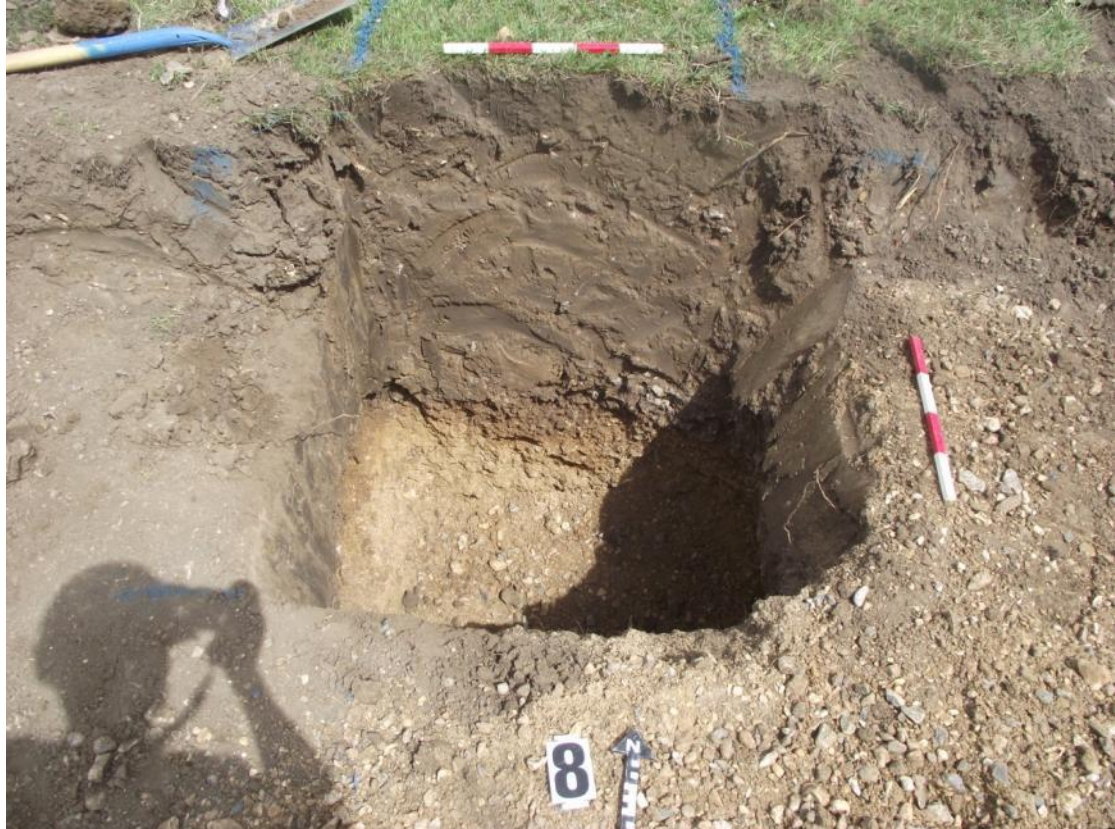
Fig 8: Saxon Primary School, Shepperton. Foundation pit 8
