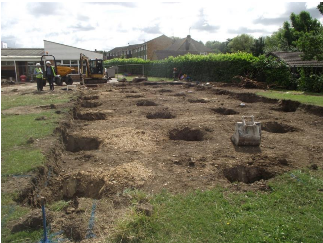
Fig 6: Saxon Primary School, Shepperton. Excavated foundation pits
