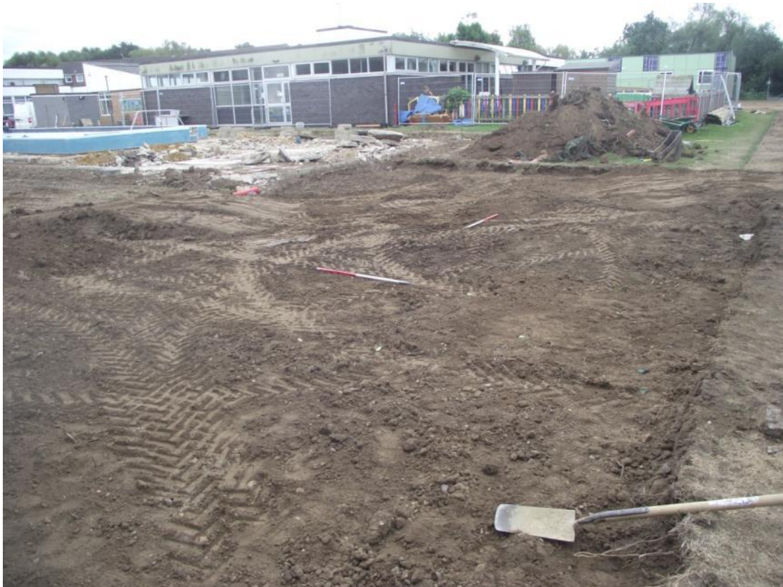
Fig 14: Saxon Primary School, Shepperton. Car park extension strip looking southeast
