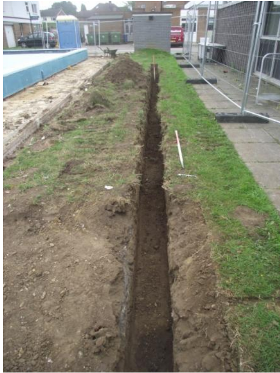
Fig 13: Saxon Primary School, Shepperton. Trench 4 (North of the nursery) looking east
