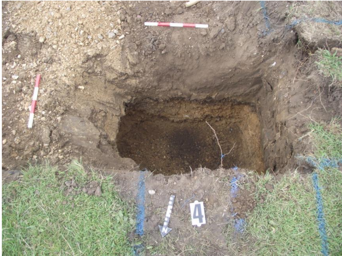
Fig 7: Saxon Primary School, Shepperton. Foundation pit 4
