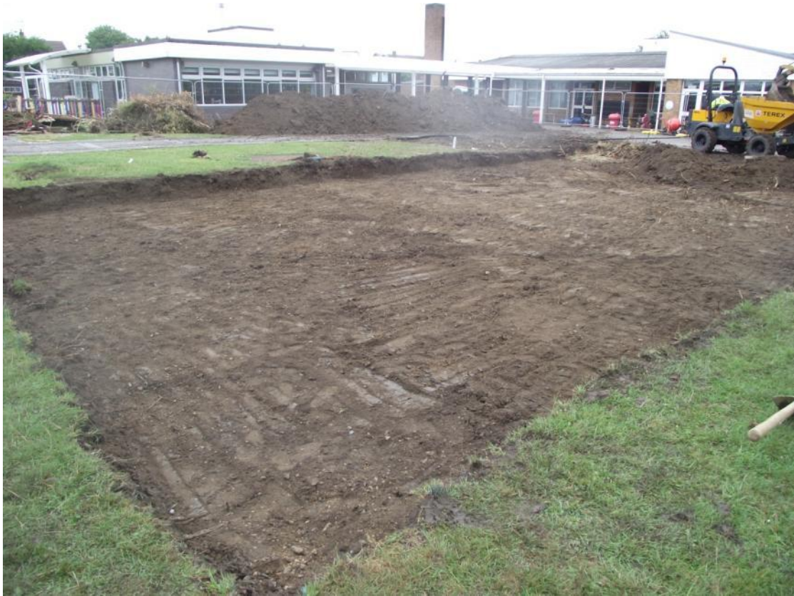
Fig 5: Saxon Primary School, Shepperton. Initial turf strip – new classroom building
