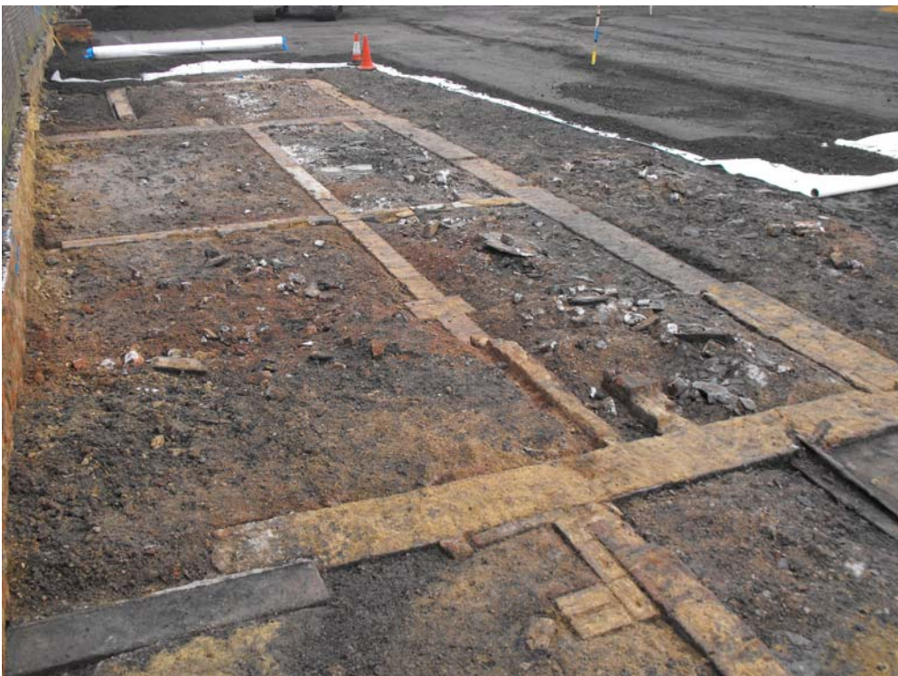
Fig 22: Looking south across building 7
