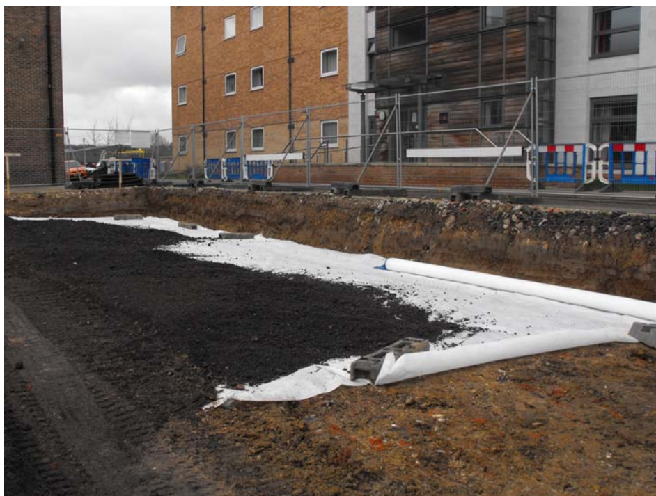
Fig 7: Area A looking south west, showing site levelling and construction
