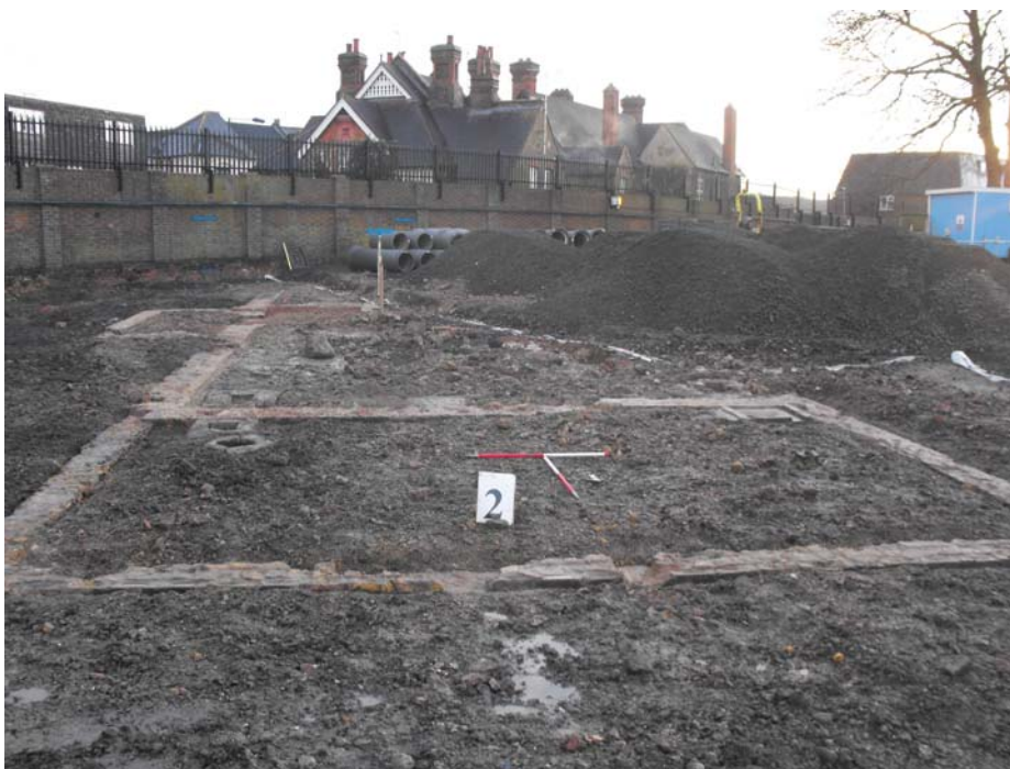
Fig 11: Looking south across building 3, showing extension (2)
