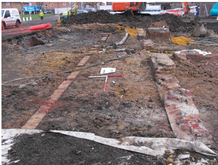
Fig 27: Looking north along A block, showing west and veranda walls, with modern disturbance
