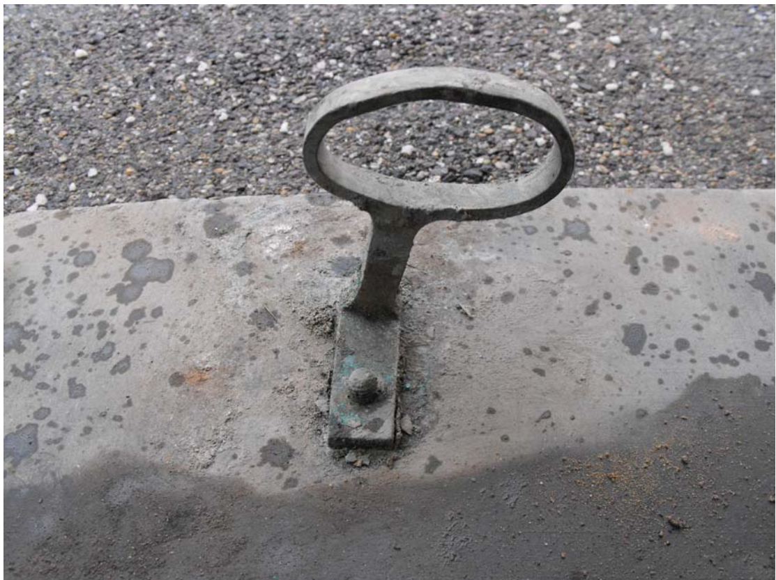
Fig 34: Detail of copper alloy fixing on slate
