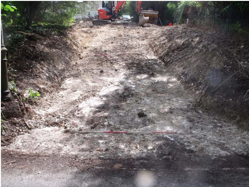
Formation level of driveway, north end, looking South
