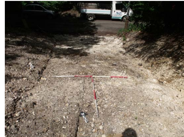
Formation level of driveway, looking north
