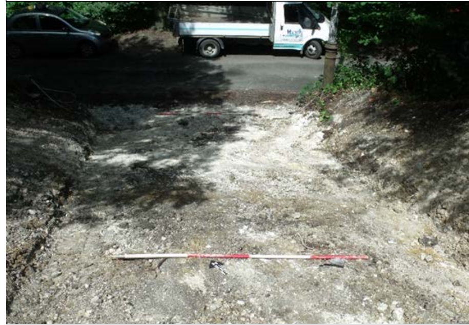
Formation level of driveway, looking north
