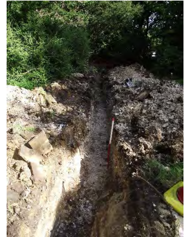
South end of trench with levelling deposit 105 in section. Looking North
