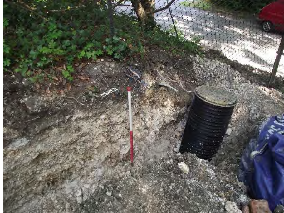
North end of pipe trench, looking north
