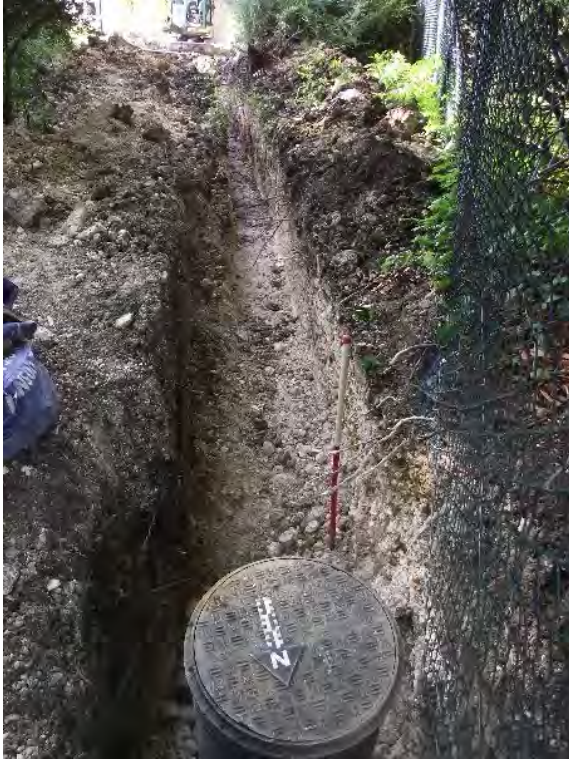
North end of pipe trench looking south
