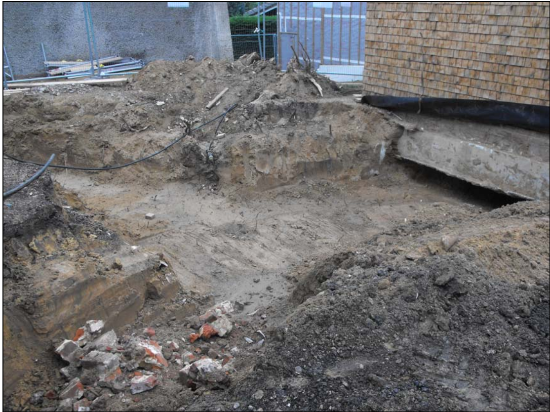
Fig 11 Area between gallery building and new build
