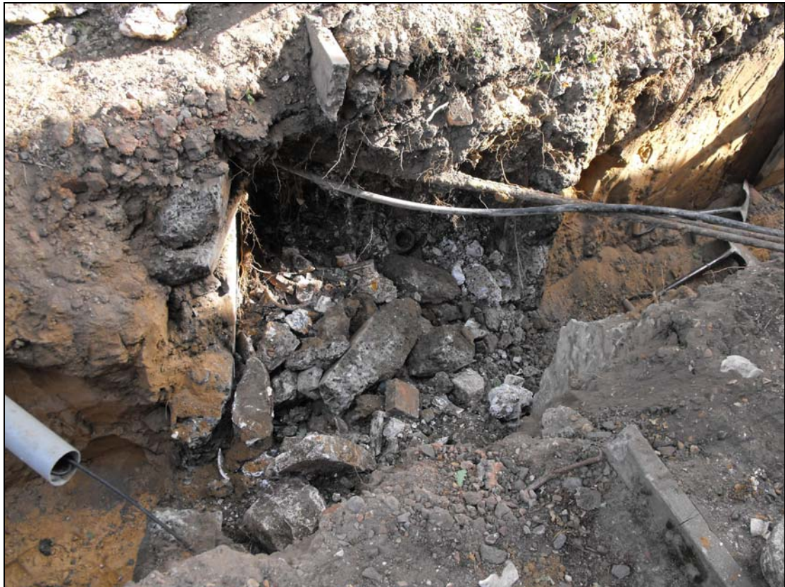
Fig 10 Culvert – western car park
