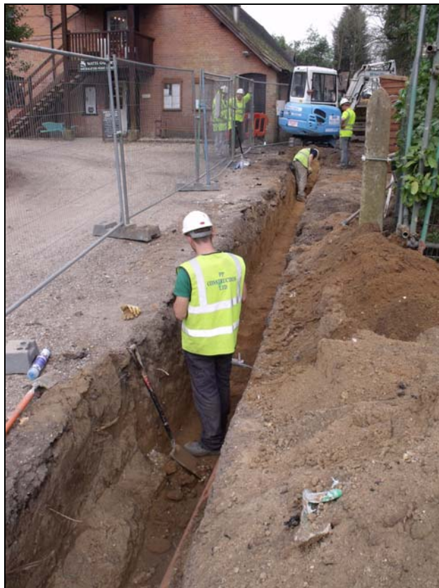
Fig 8 Long drainage trench – Old Kiln
