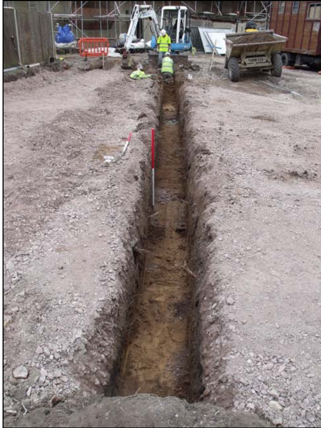
Fig 7 Service trench three – western car park
