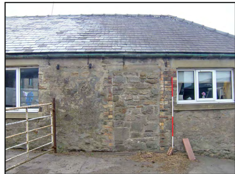
Photo 16: The north end of the east elevation of the east range.
