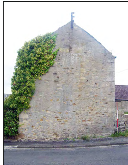
Photo 04: The west elevation of the south range.
