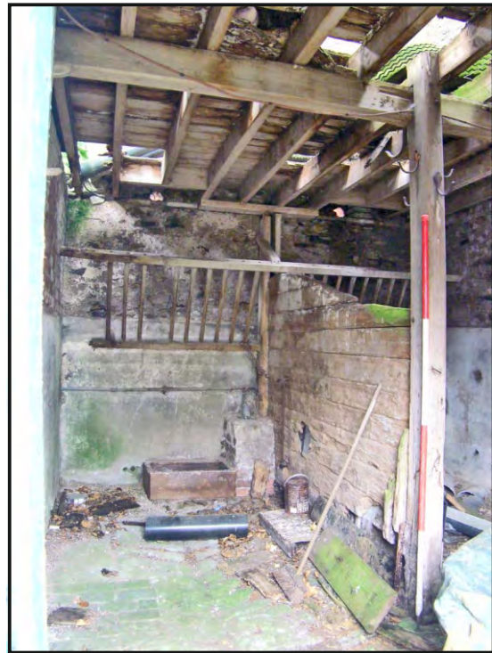
Photo 22: Internal view of the west compartment of the south range.
