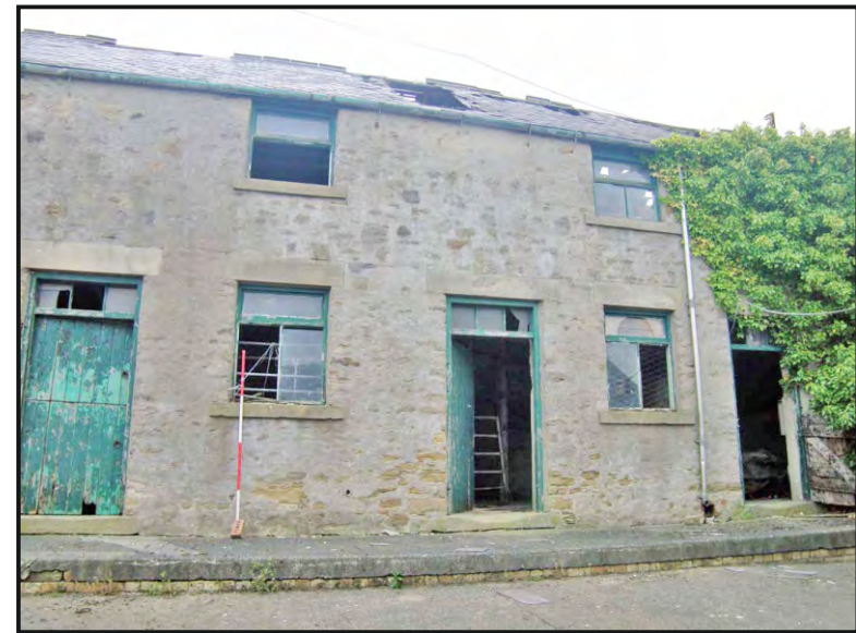
Photo 20: The west part of the north elevation of the south range.
