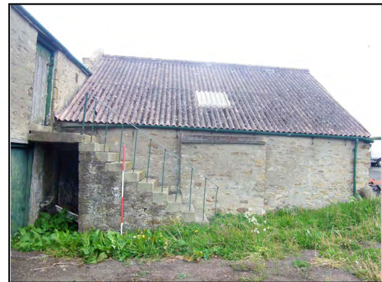
Photo 08: Steps to first floor granary built against the west elevation of the attached south-east building.
