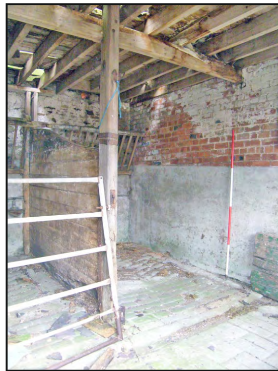
Photo 24: View SW into the west-central compartment of the south range.
