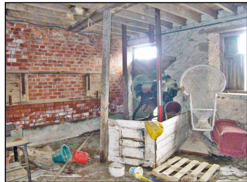
Illus. 28: View north-westwards from the SE corner of the east compartment of the south range, showing blocked openings in the dividing wall and rolling machine to centre of view.
