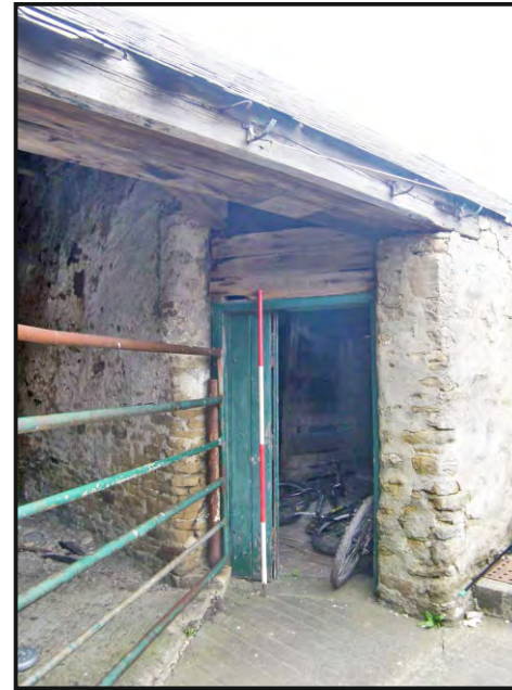
Photo 18: Doorway into the central compartment of the east range.
