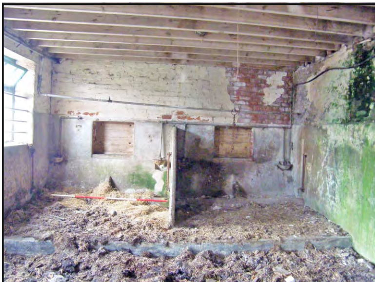
Photo. 27: View of the east wall of the east-central compartment of the south range, showing stall division and blocked openings.
