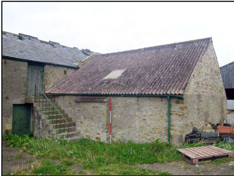
Photo 09: View of the south-east building from the south-west side.
