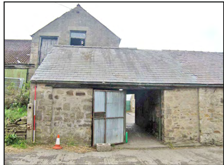
Photo 14: The south end of the east elevation of the east range.
