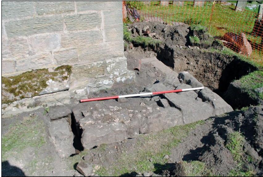
Illus. 45: View looking east across completed excavation of Tower foundations adjacent to the southwest corner of the Nave.
