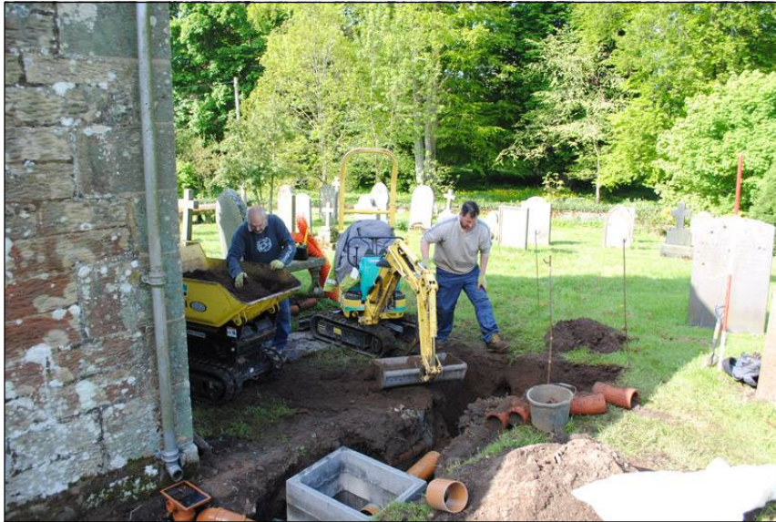
Illus. 27: View looking southwest at excavation of services trench and soak-away pit, adjacent to the northwest corner of the nave.
