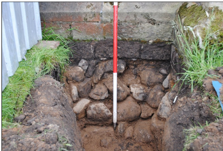
Illus. 23: Detailed view of north-facing section in Trench 2, showing dry-stone cobble foundation raft.
