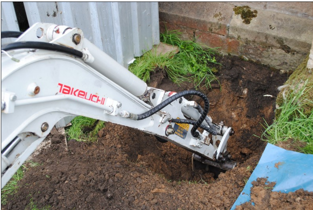
Illus. 20: Detailed view looking southeast during the excavation of Trench 2.
