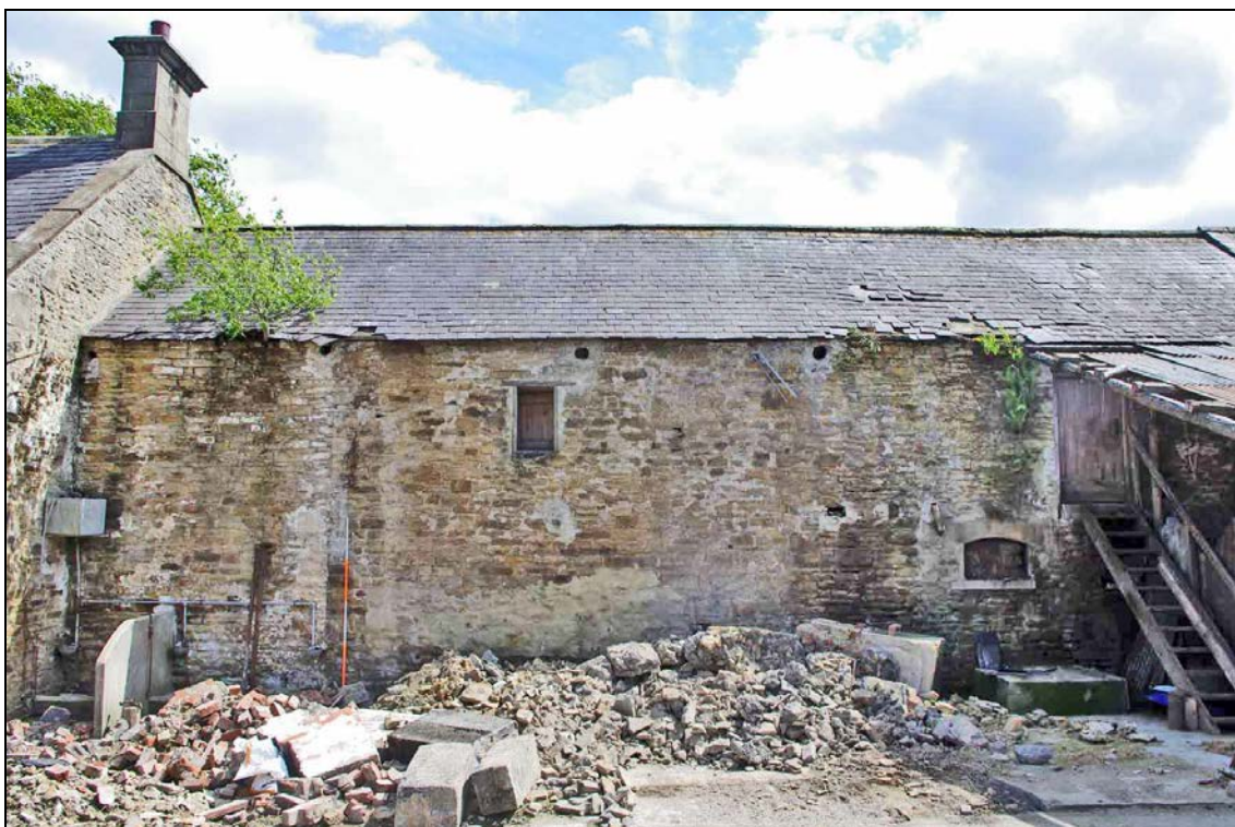
Frontispiece: North elevation of the east part of the Main Range.
