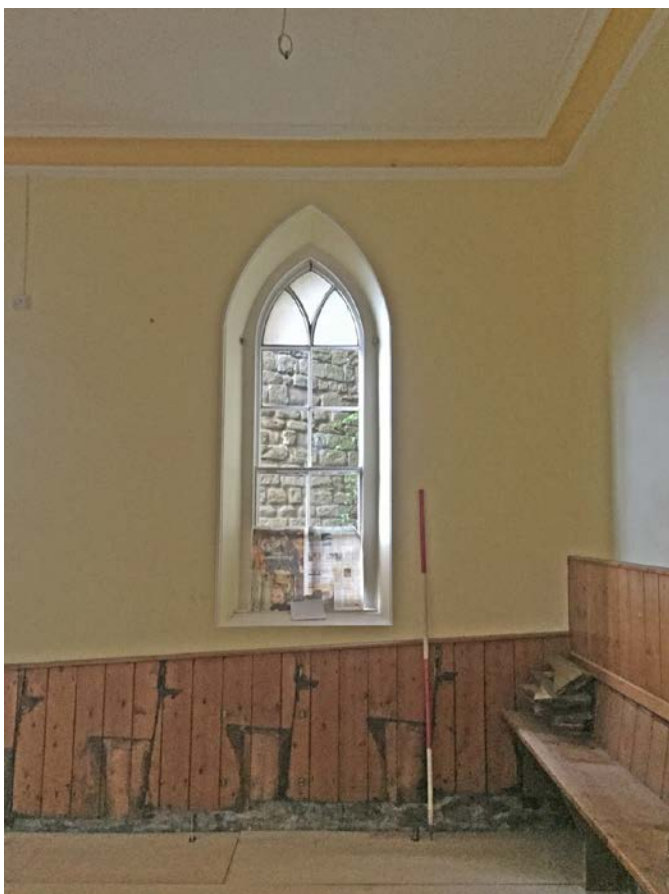
05: Window in the north-west wall.
