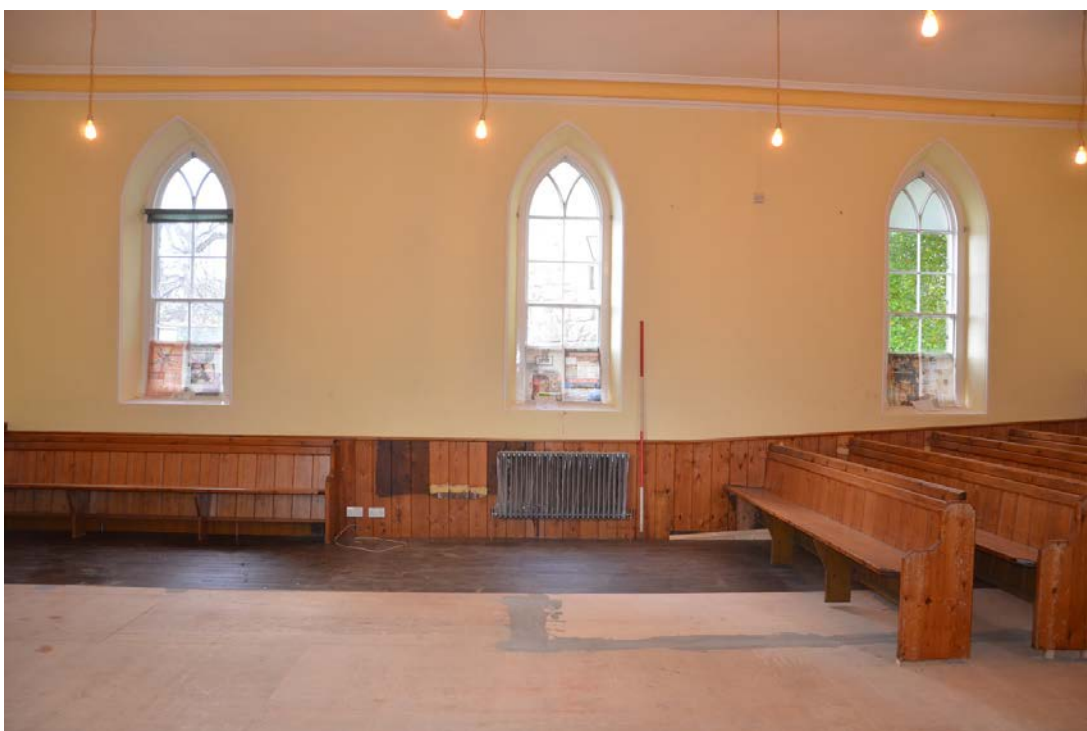
04: The inner face of the north-west wall.
