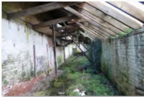
19 E Range Outshut looking N
