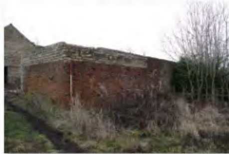
131 Wall W of N entry
