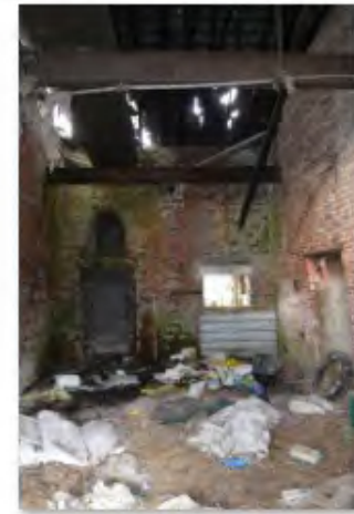
123 Engine Ho looking N
