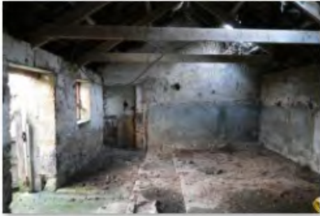
82 S Range W compartment looking E
