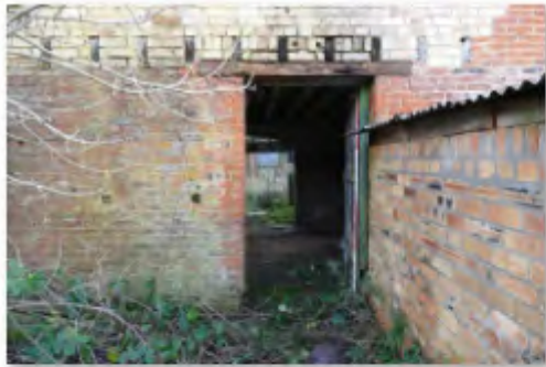
55 Centre Range door at E end
