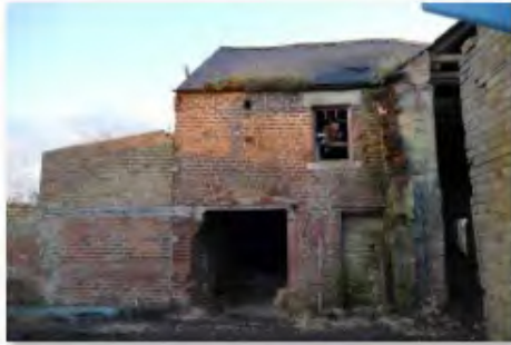
109 Engine House from S
