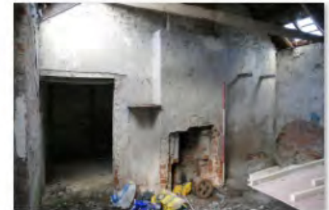
72 SE Range S compartment looking NE
