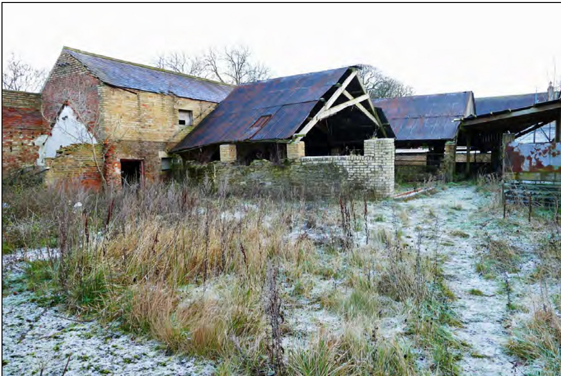
Illus. 25: The Covered Yards, viewed from the north-west.
