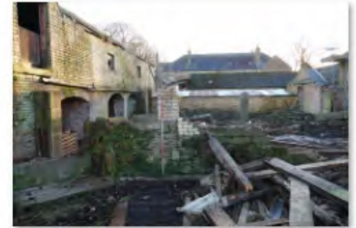
48 Centre Range N side
