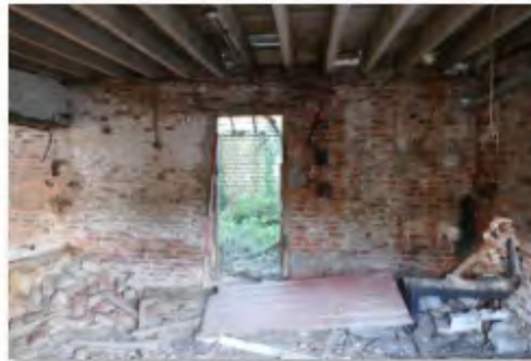
50 E Range centre compartment looking E
