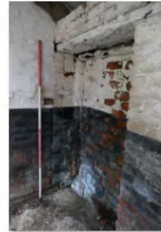
93 W Range S part blocked door on W
