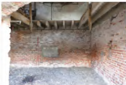
52 E Range centre S compartment looking E
