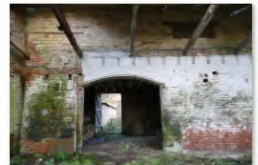
18 E Range Outshut S end looking W
