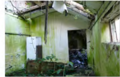
24 E Range Outshut centre of N rooms looking N
