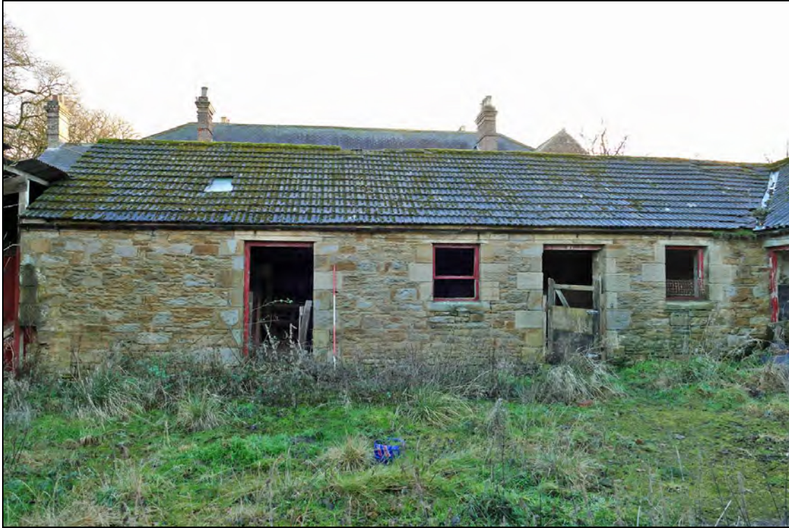
Illus. 18: The South Range viewed from the north.
