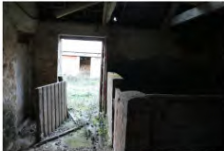
80 S Range E compartment looking N
