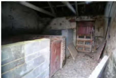
79 S Range E compartment looking S
