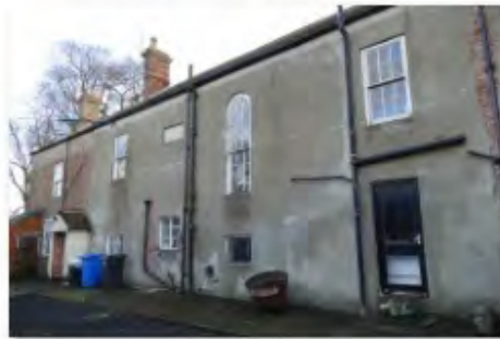
140 House north frontage from the NW _
