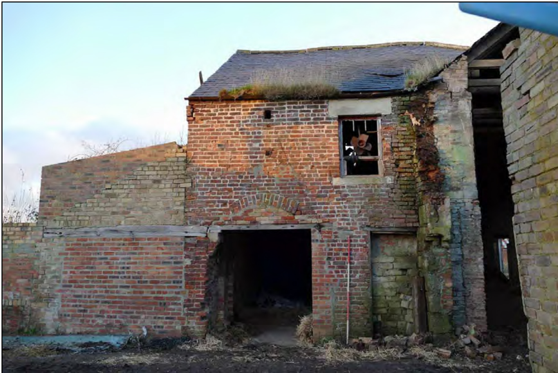
Illus. 21: The Engine House, viewed from the south.
