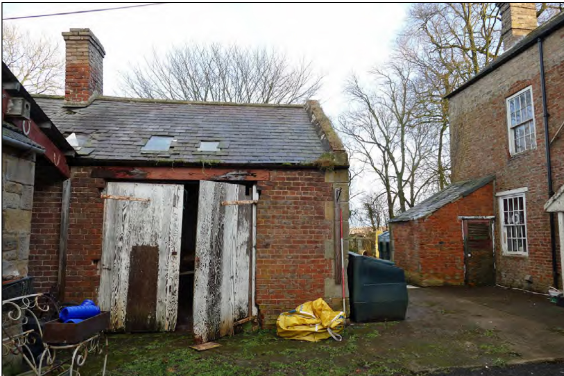
Illus. 24: The South-East Range, south part viewed from the west.
