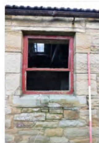
81 S Range N centre window
