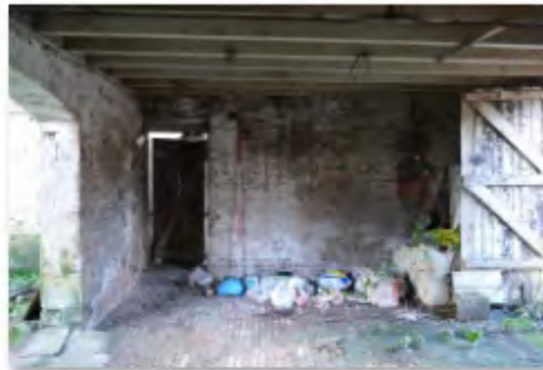
56 E Range S compartment looking S
