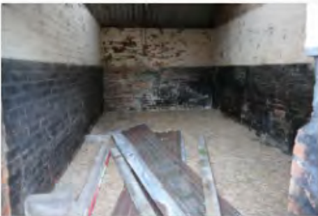
94 W Range S part Nmost compartment looking W
