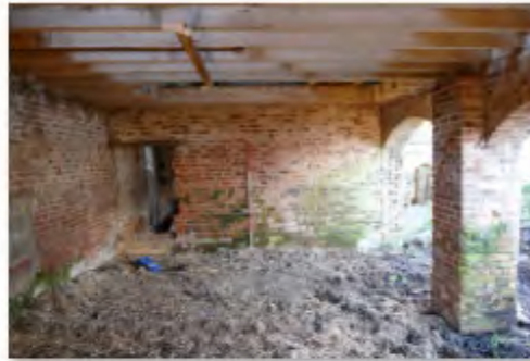
47 E Range centre N compartment looking S
