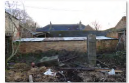
57 Centre Range looking S
