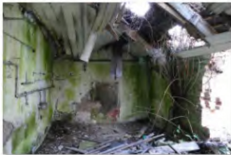
25 E Range Outshut N of N rooms looking N
