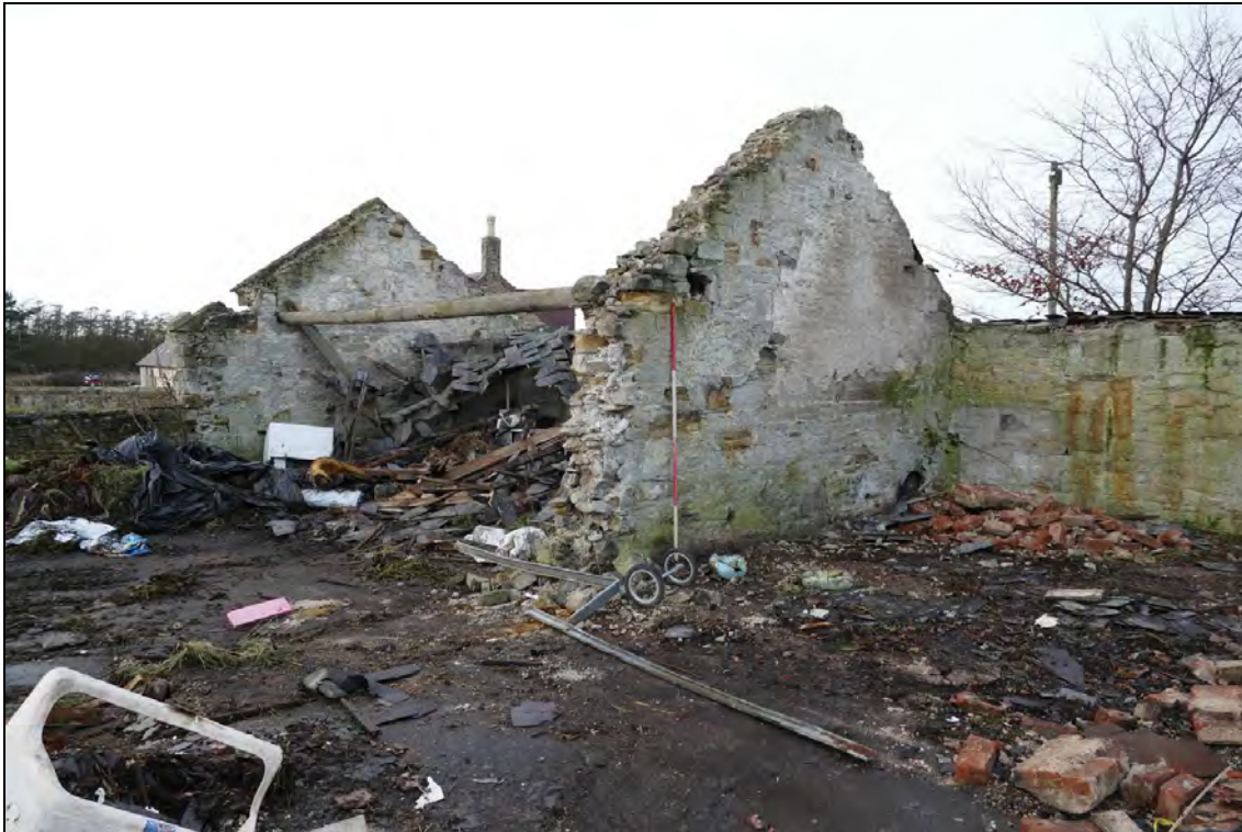
Illus. 27: The North-West Range, viewed from the south-east.
