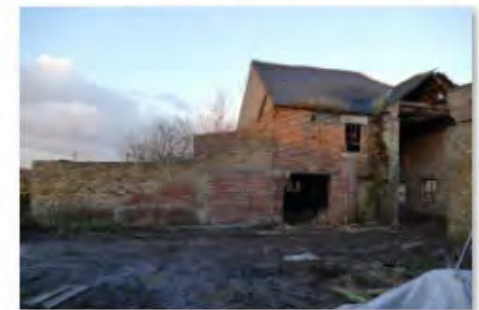
108 Engine House from SSW
