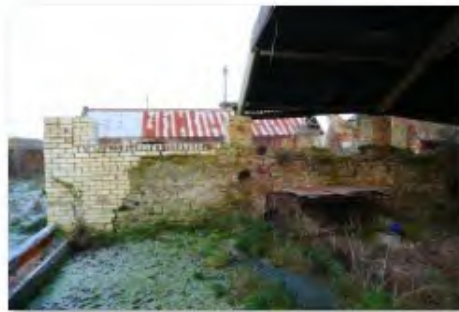
137 N covered yard looking N
