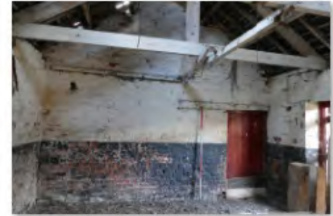
75 SE Range N compartment looking SW
