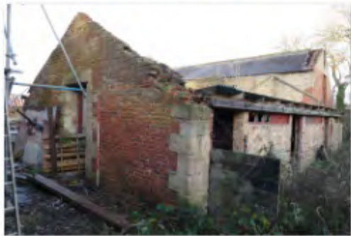
58 Centre Range from SW
