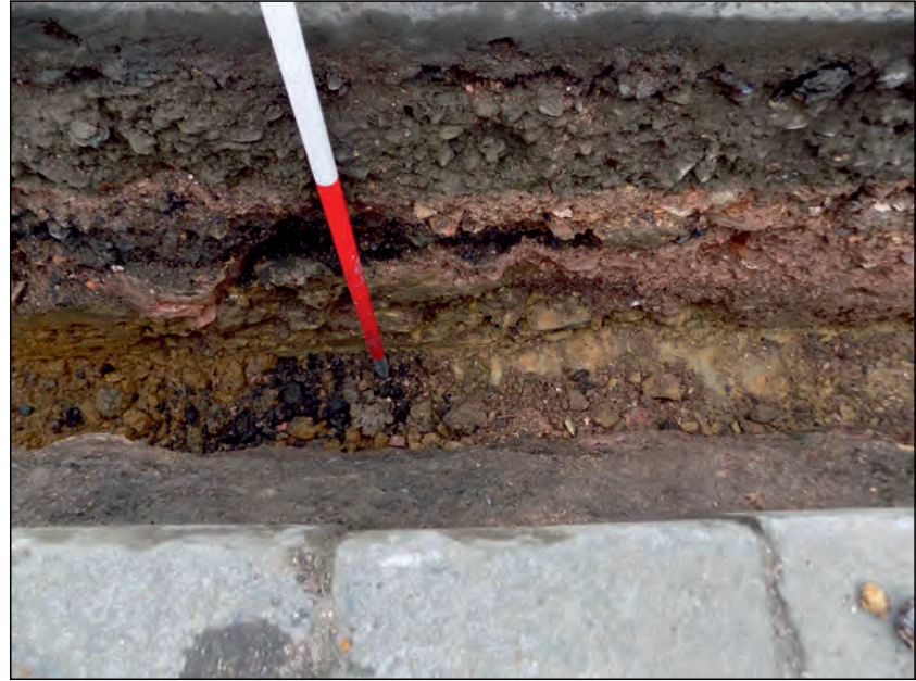
Photo 6. South facing section of cable trench, located approx 17m from start of trench.
