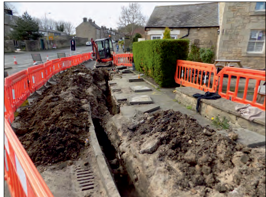
Photo 4. General working shot during cable trenching, view looking WSW.
