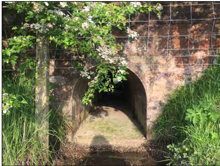
Frontispiece: View of culvert on the east side of the site.
