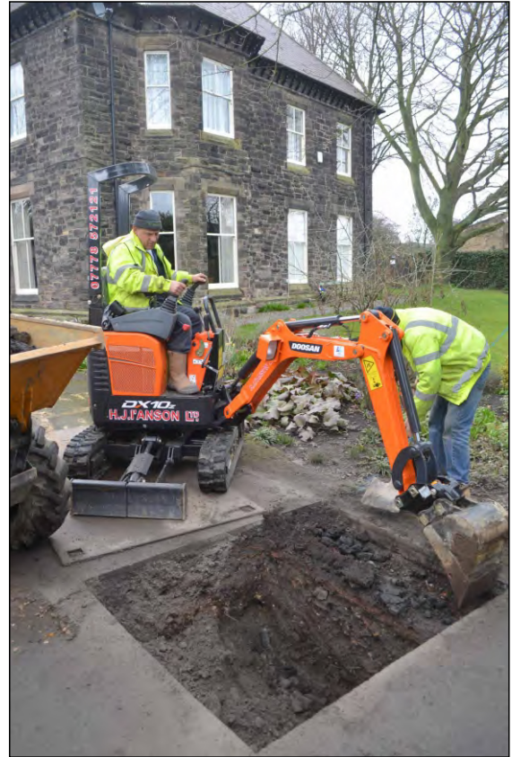
Photo 73. View looking NE during excavation for new manhole under Vicarage Driveway.
