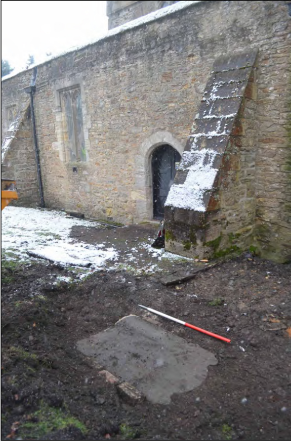
Photo 27. Reused grave-marker, covering a soak-away drain [03] near western buttress.
