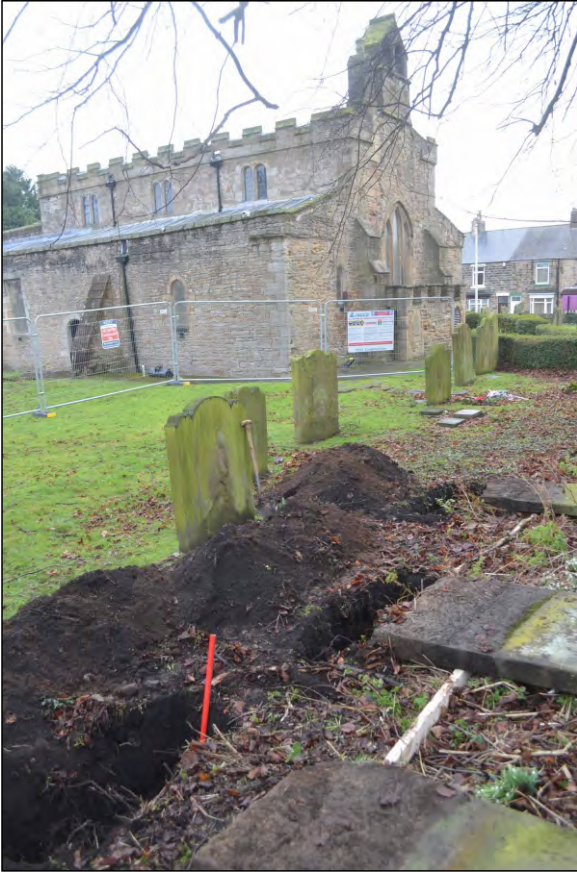
Photo 23. Third slot excavated for relocated grave-marker.
