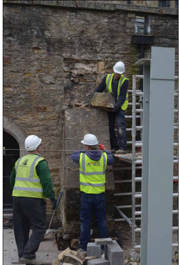
Photo 87. The western buttress during further removal of upper courses.
