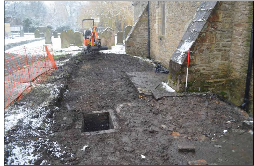
Photo 32. Clearing turf from the extension area revealed a brick soak-away drainage tank [03]. View looking east.
