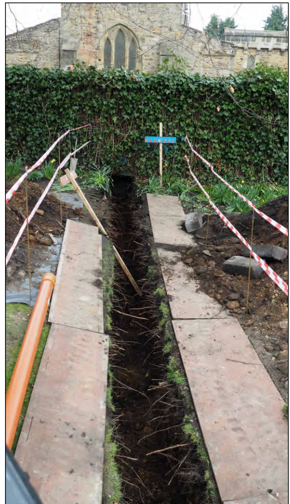
Photo 75. View looking east along services trench excavated in Vicarage lawn.
