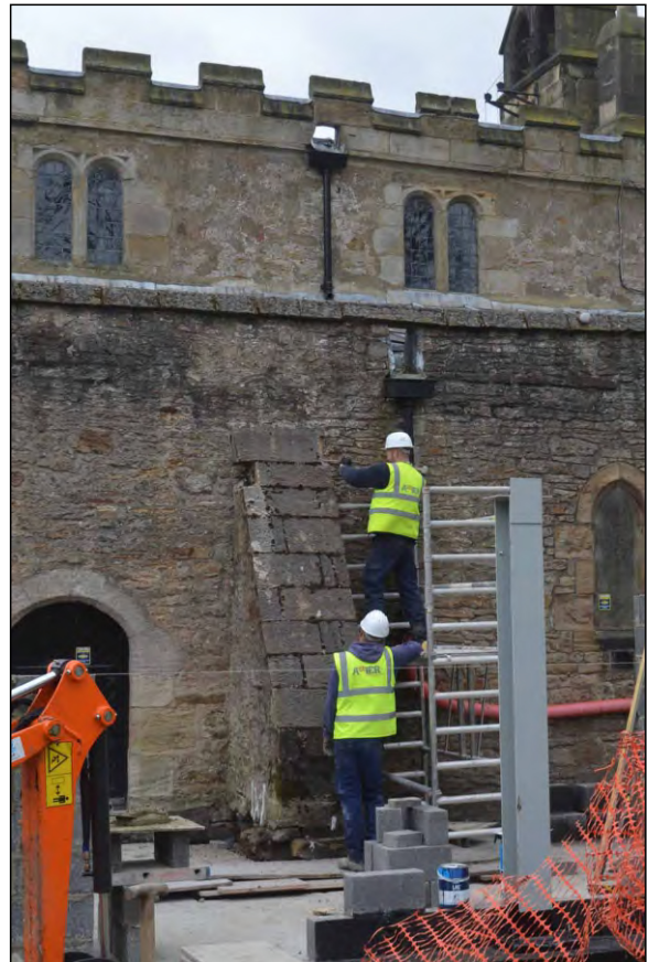
Photo 85. The western buttress at the beginning of reduction works.
