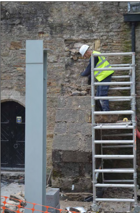
Photo 88. The western buttress during final removal of upper courses.
