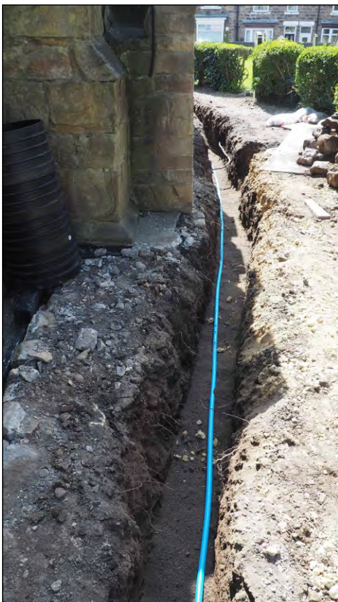
Photo 78. View looking south along services trench at east end of Church.
