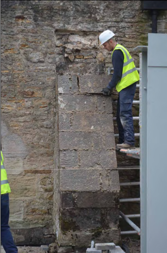
Photo 86. The western buttress during removal of upper courses.
