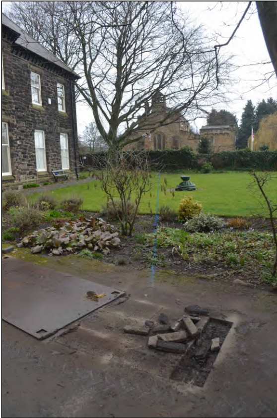
Photo 72. View looking east during excavation for new manhole under Vicarage Driveway.
