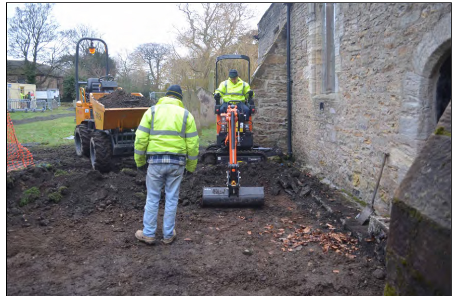
Photo 42. Further excavation in the central area of extension.
