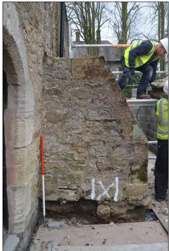
Photo 89. The western buttress after removal of upper courses.
