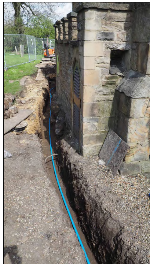
Photo 79. View looking north along services trench at east end of Church.
