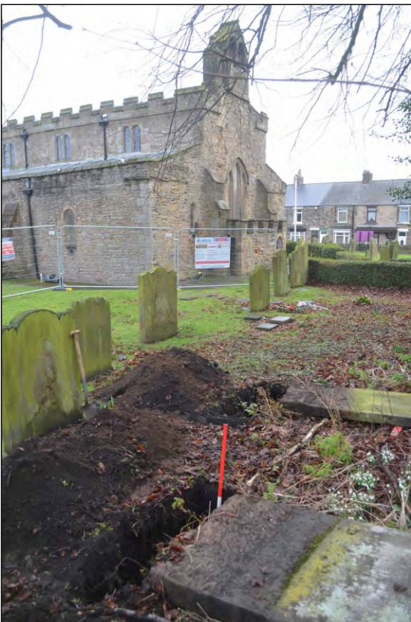
Photo 21. Second slot excavated for relocated grave-marker.
