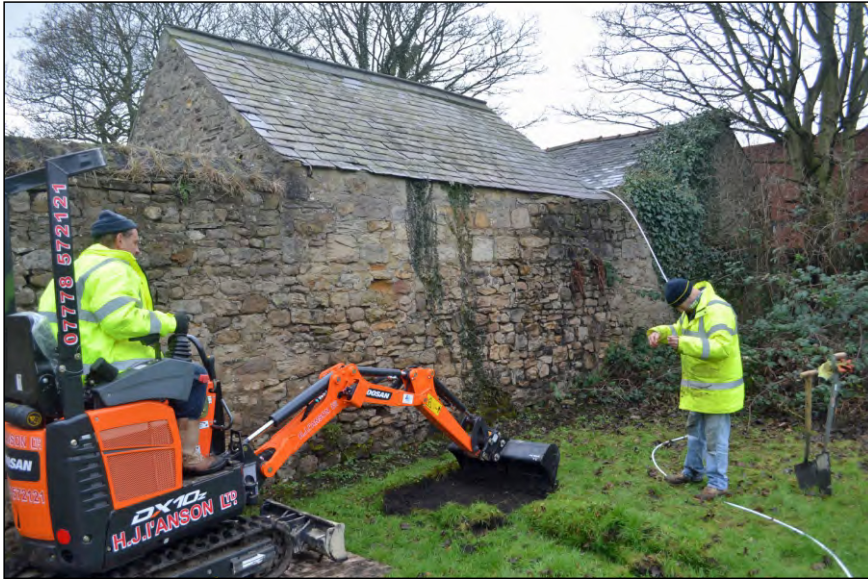
Photo 69. View looking SW during excavation of new charnel pit [06] to house disarticulated bones uncovered in extension area.
