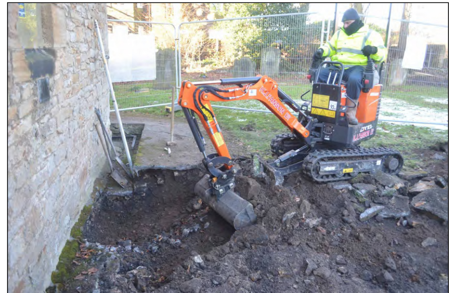
Photo 34. View looking west during excavations for new extension.
