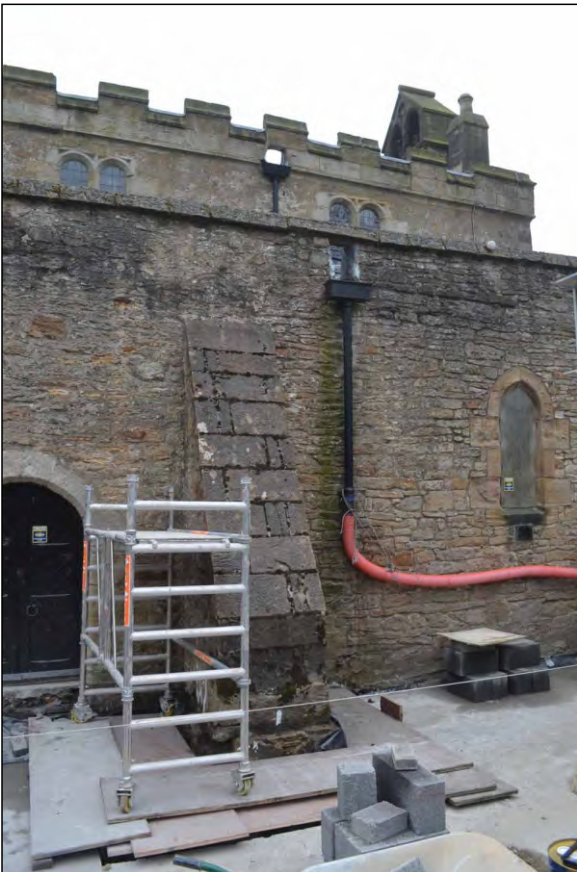
Photo 84. The western buttress prior to reduction.
