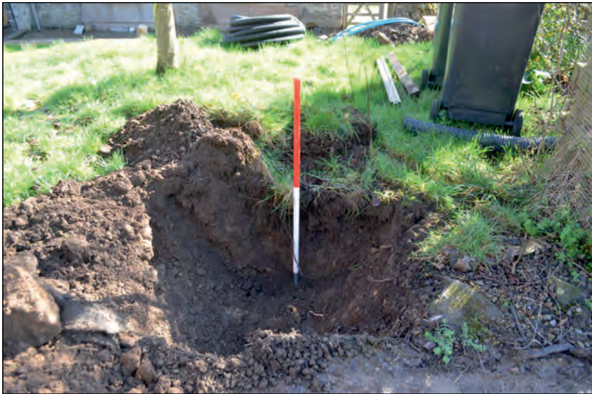
Photo 11. View looking east-southeast at small trench for Gatepost 4.
