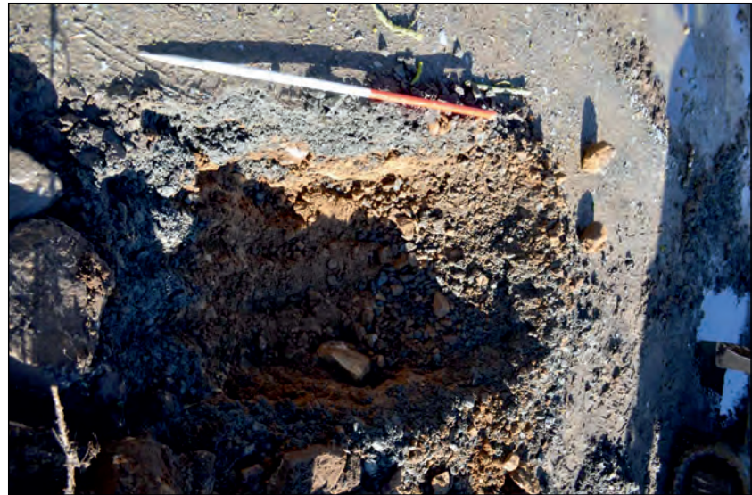
Photo 8. View looking north-northeast at small trench for Gatepost 2.
