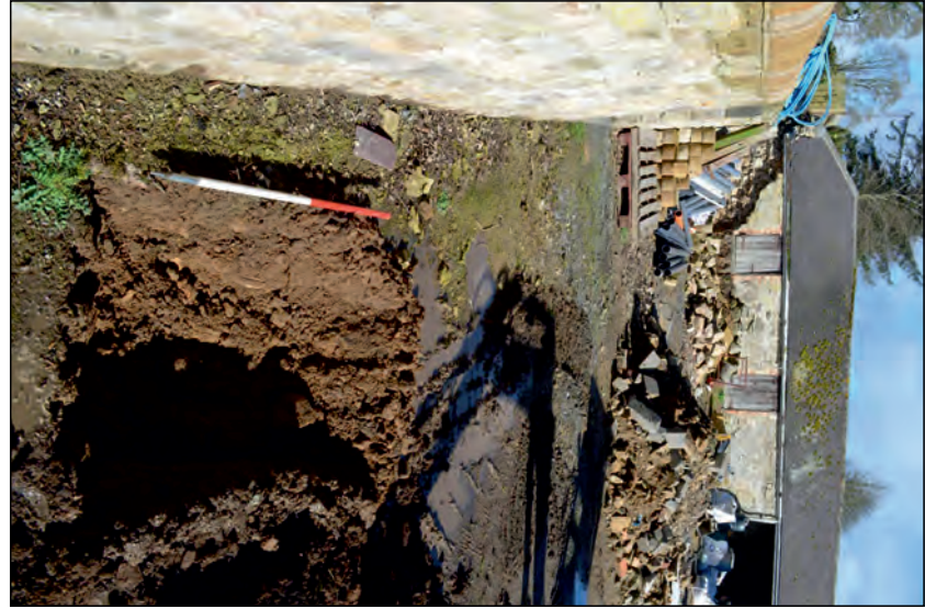
Photo 6. View looking north-northeast at small trench for Gatepost 1.
