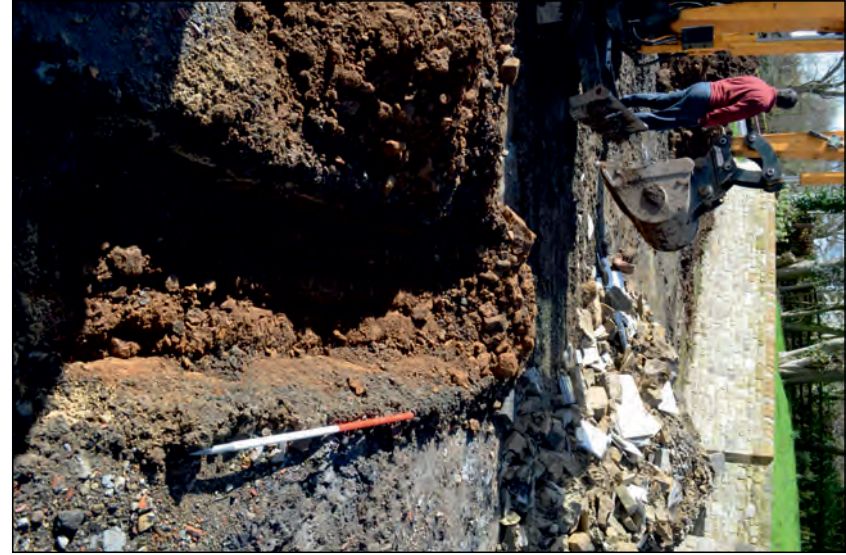
Photo 14. View looking west-southwest along of portion of property boundary fenceline trench and driveway area.
