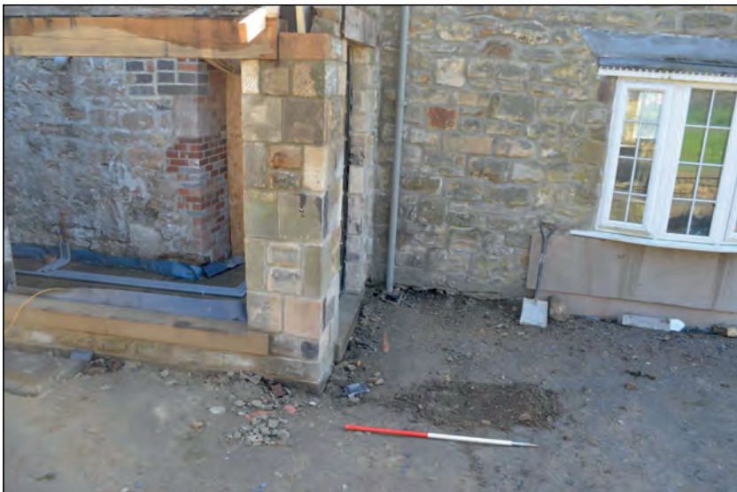
Photo 19. View looking east-southeast at post-pad location for new porch timber.
