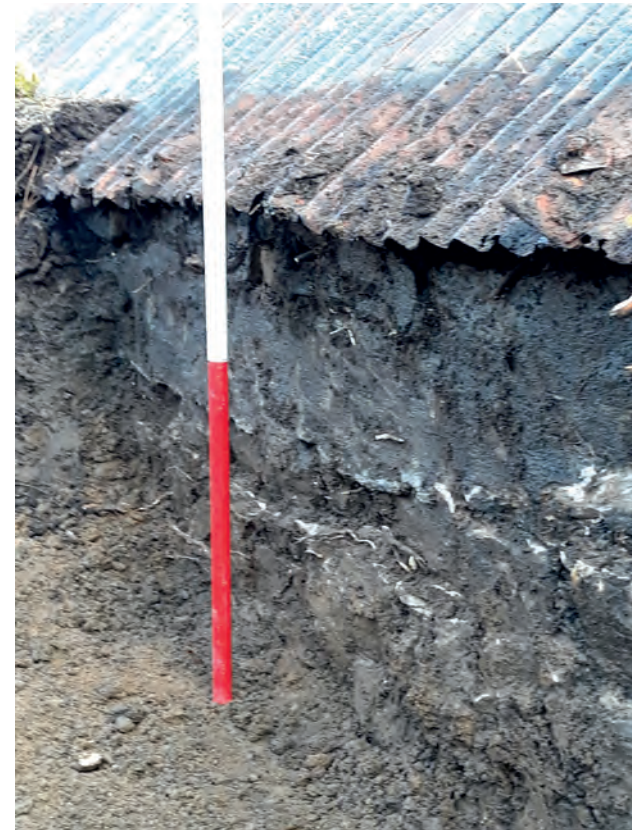
Photo 06: West wall of byre, showing sandstone construction underlying rendered upper level
