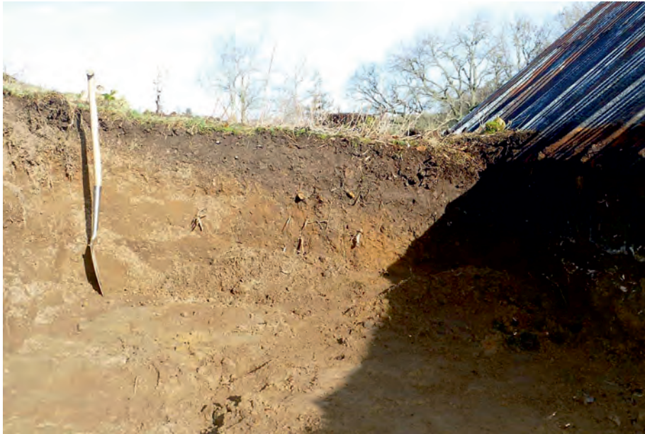
Photo 04: South facing section behind west wall of byre, showing soil creep and silting against the wall and roof of the building
