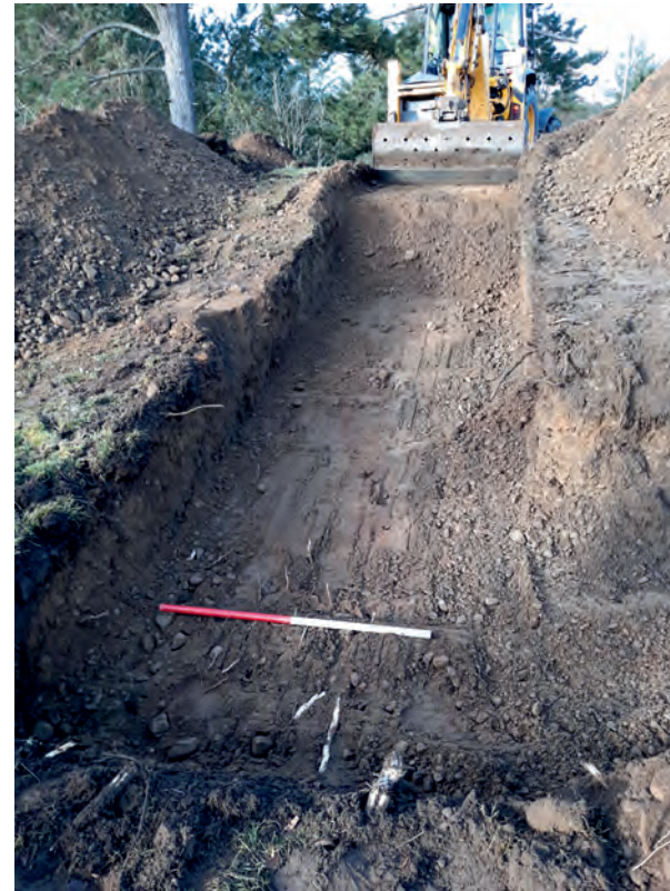
Photo 03: East-west arm of trench running up glacial mound, looking west
