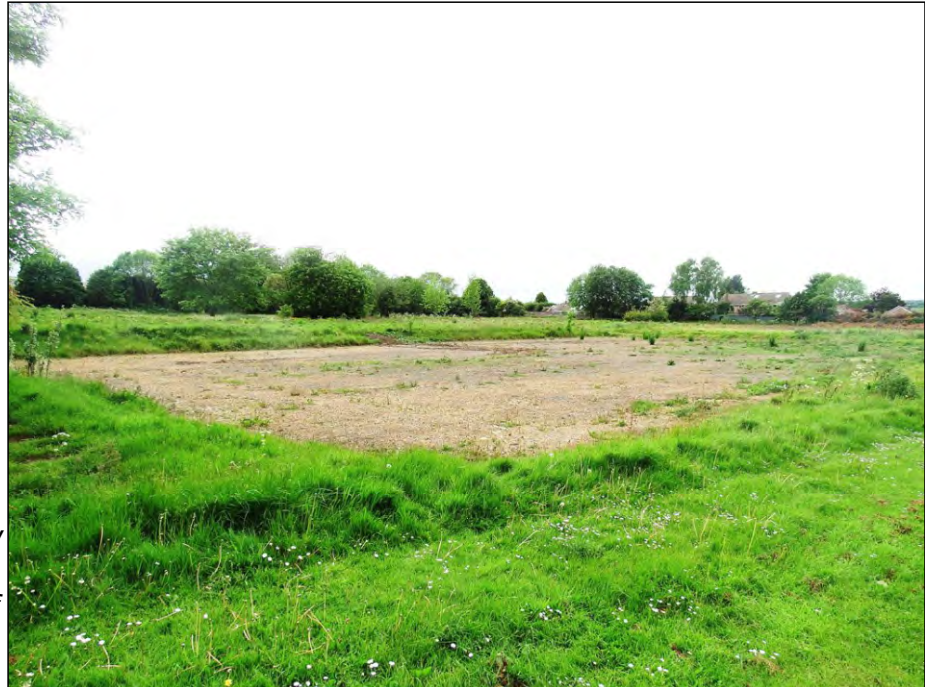
Photo 8: Looking SW from the NE corner over the site of one of the demolished college buildings.
