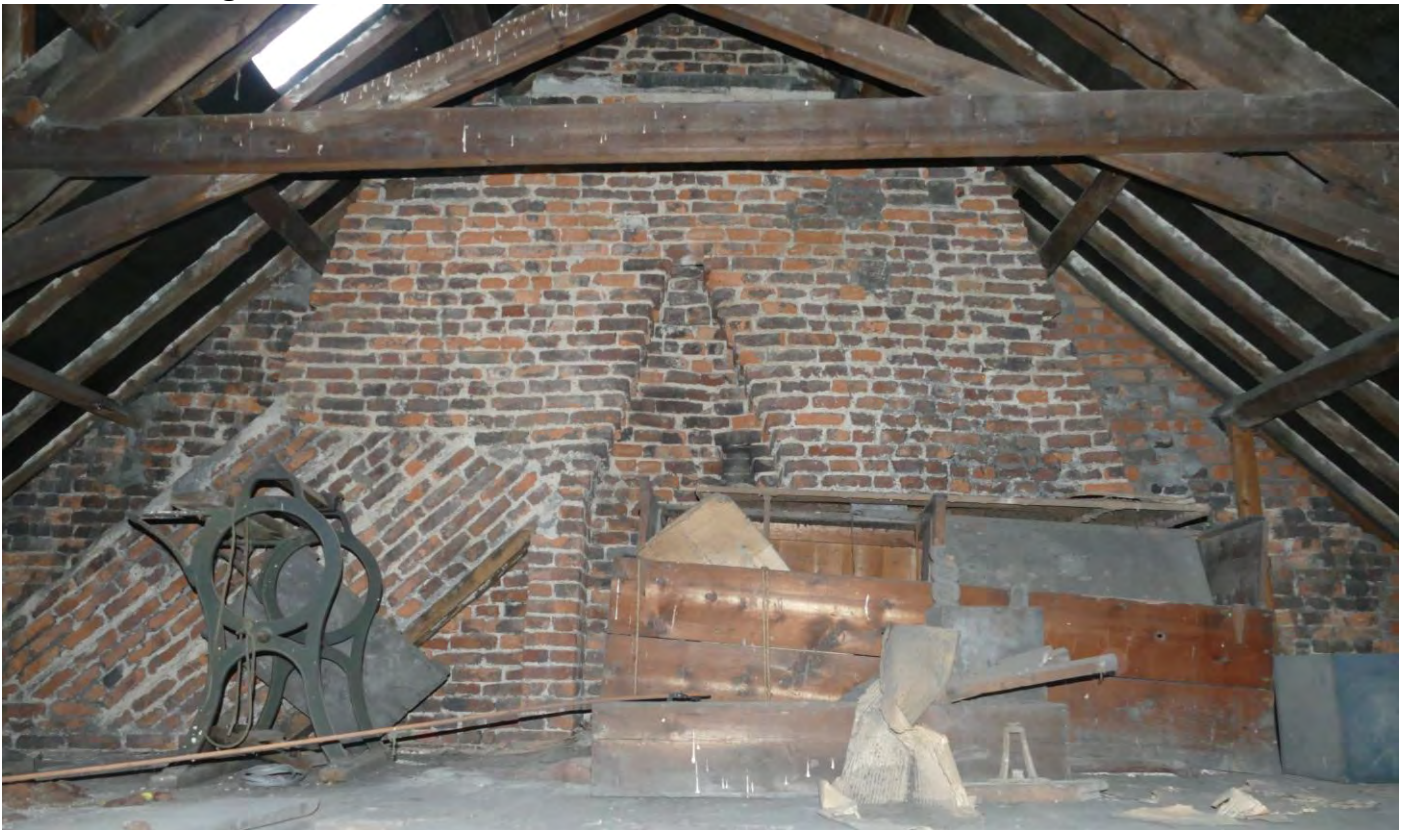
Main Block attic looking north
