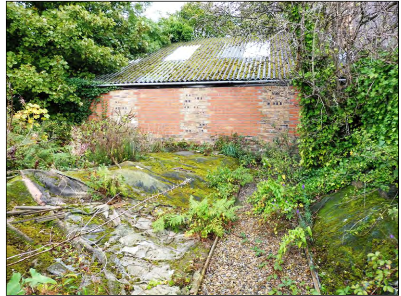
Photo 14: View of the open area looking N towards rear wing building 5.
