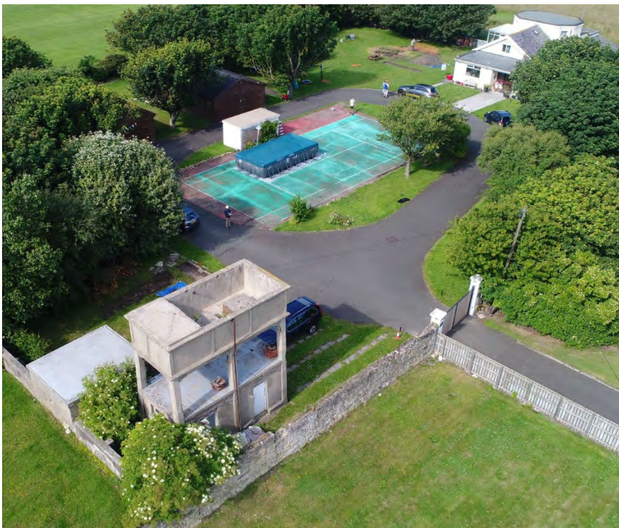
Illus. 06: View of the site from the south- west during excavations
