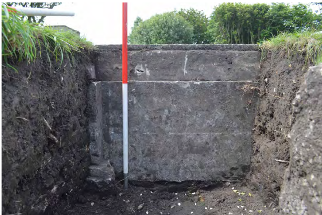
Illus. 35: Trench 8, showing concrete wall
