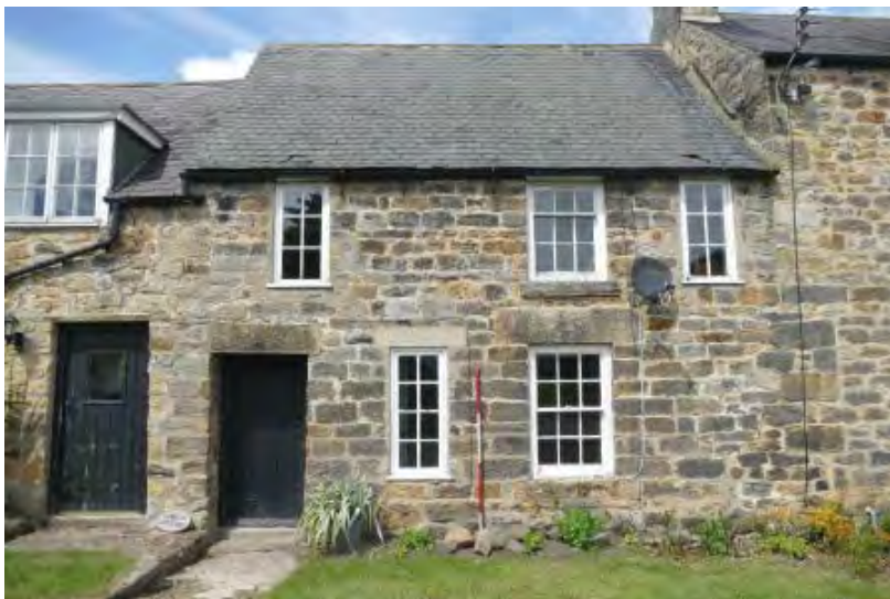
Illus. 08: South elevation of the east part of the cottage.
