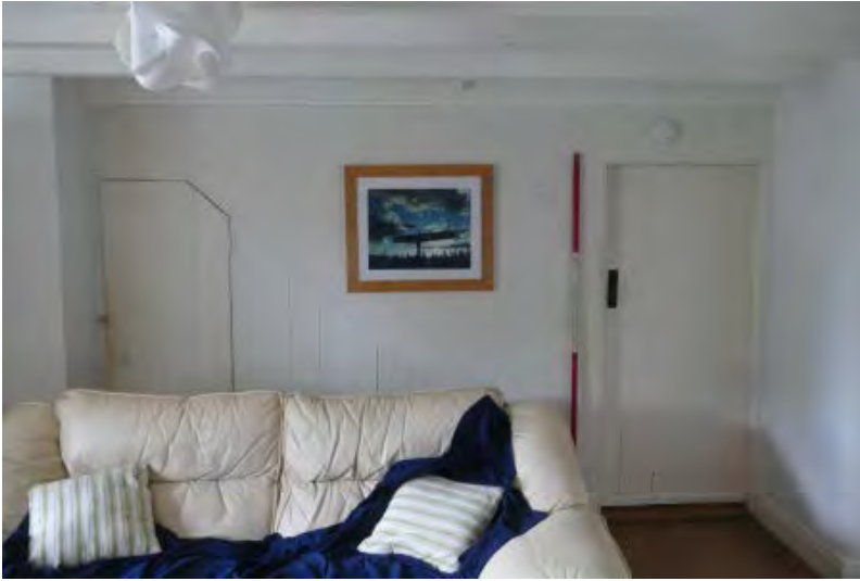
Illus. 10: boarded partition between GF living room and stair.
