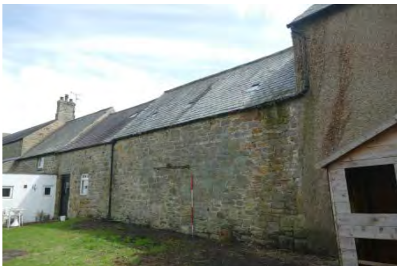
Illus. 09: The north elevation viewed from the north-west.
