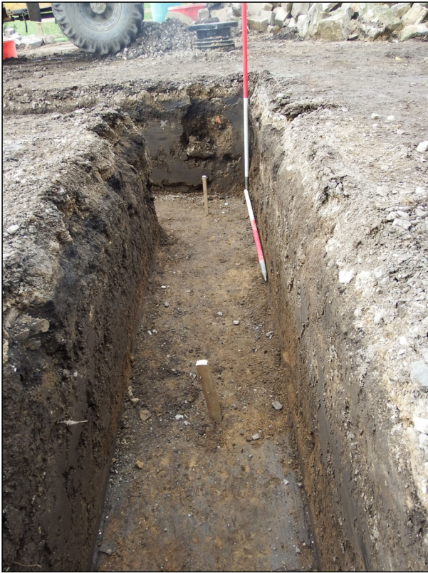
Photo 5: View looking WNW along north foundation trench.
