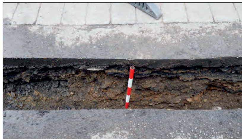
Photo 34. Area B13, south facing section.
