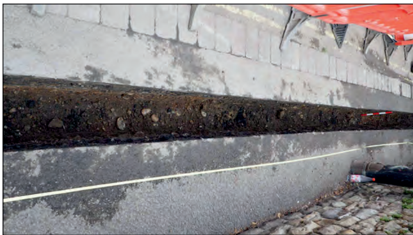
Photo 33. Area B13, view looking east.
