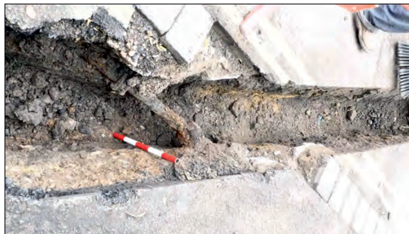
Photo 42. Area B18, view looking ENE at modern pipe.
