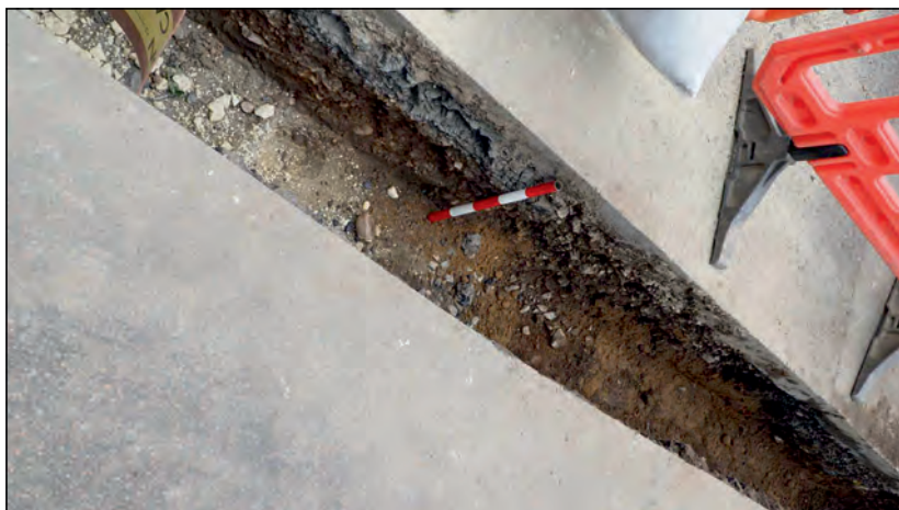
Photo 29. Area B9, view looking east.
