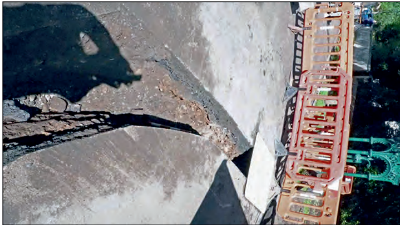
Photo 3. Area B0, looking north.
