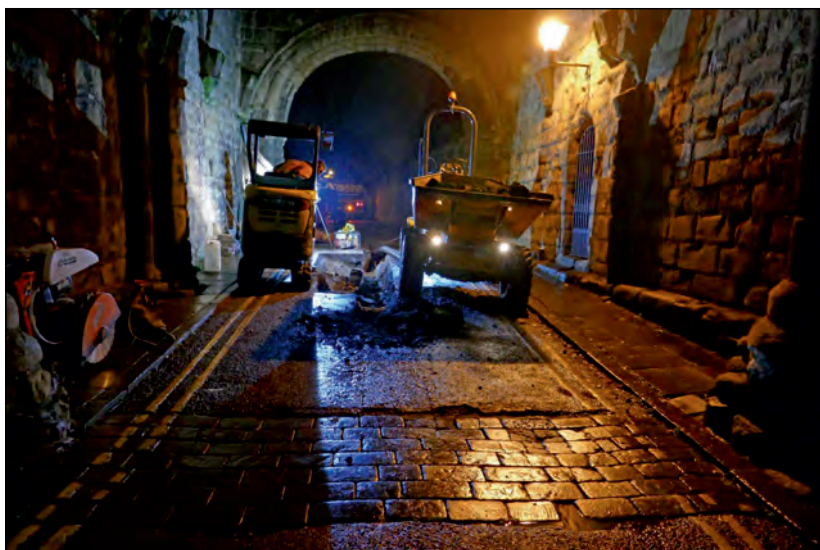
Photo 59. Area D2, view looking SSW.
