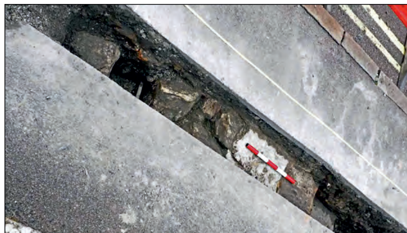
Photo 52. Area C2, view looking WNW at detail of masonry [13].
