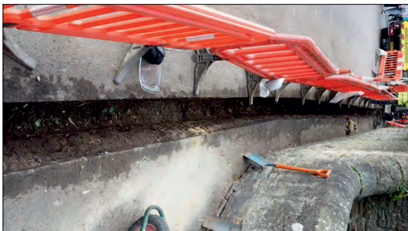
Photo 39. Area B16, view looking east.
