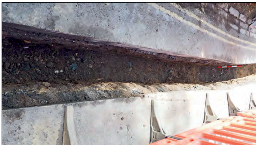
Photo 25. Area B7, view looking WNW.
