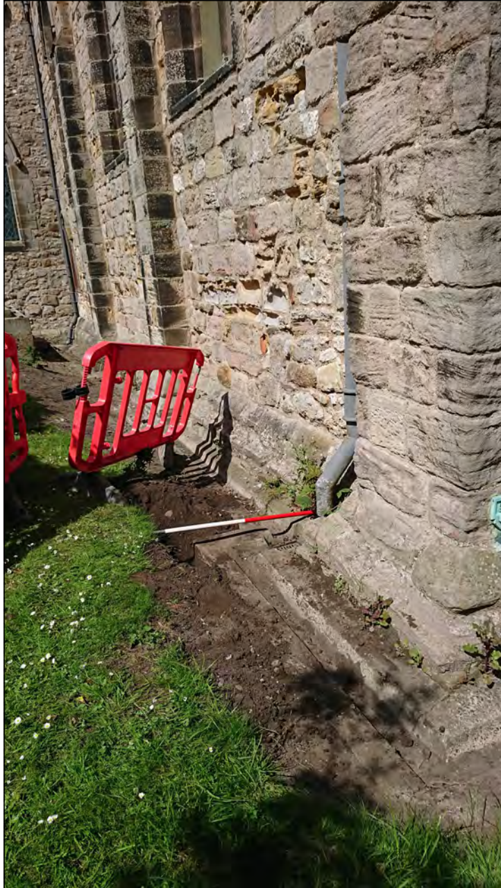
Photo 05. Broad view looking west towards Drainage excavation GY05.
