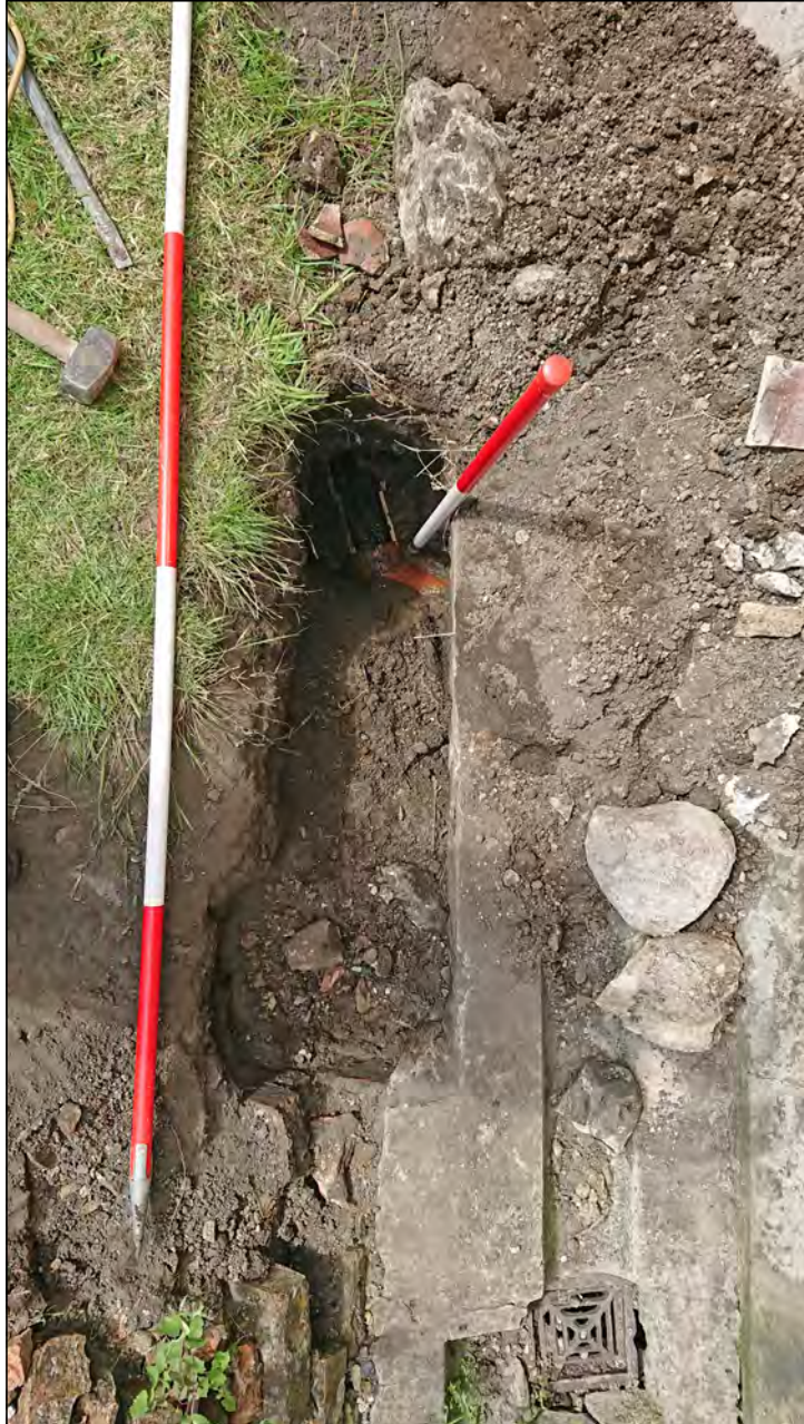
Photo 11. View looking west along Drainage excavation GY07.
