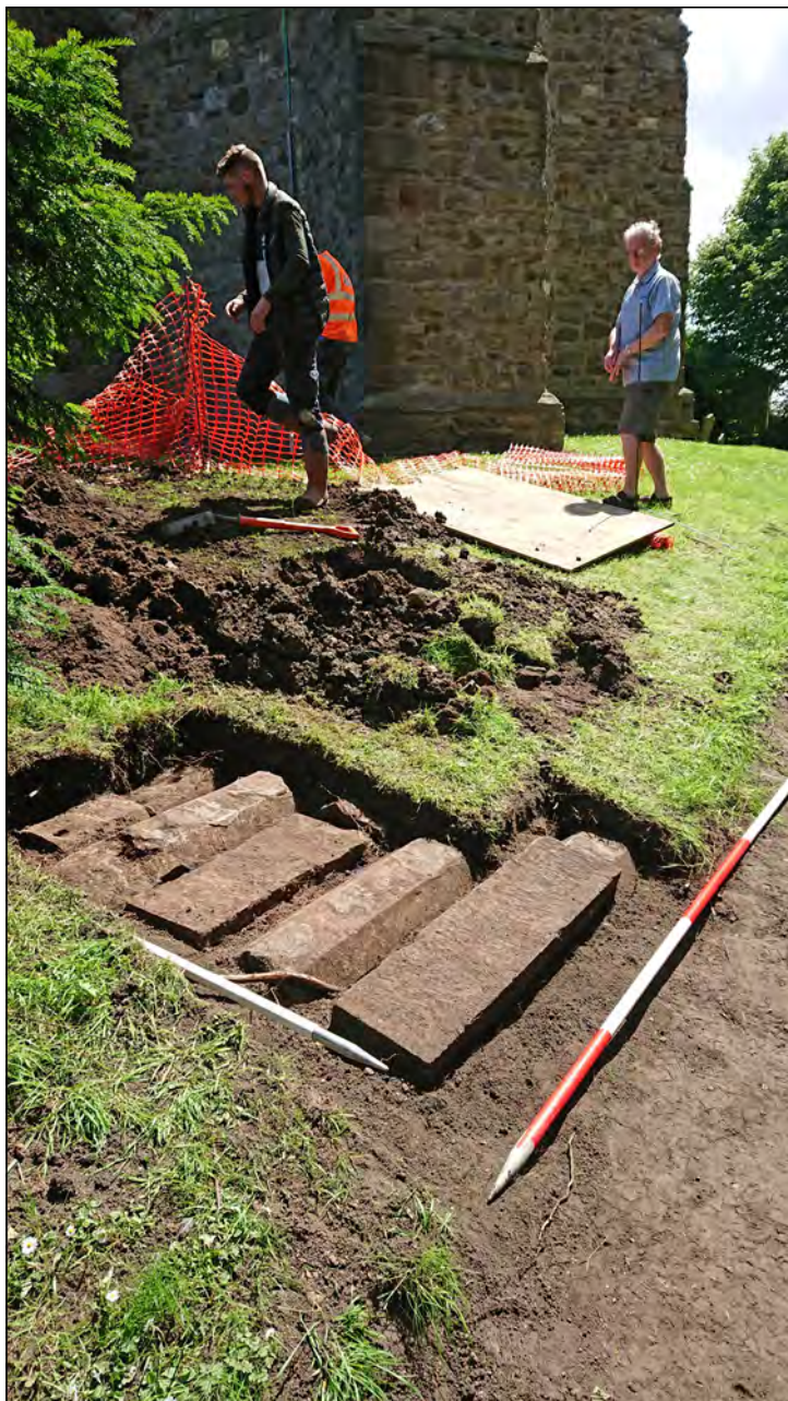
Photo 16. Broad view looking southeast, showing a row of stone slabs reused probably in the 20th century torevet the main pathway retaining wall.
