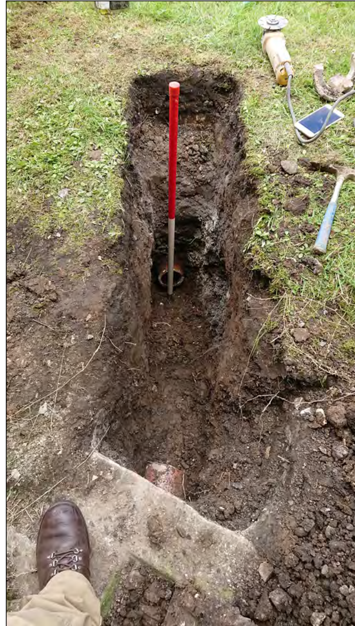
Photo 04. View looking northwest along Drainage excavation GY02.
