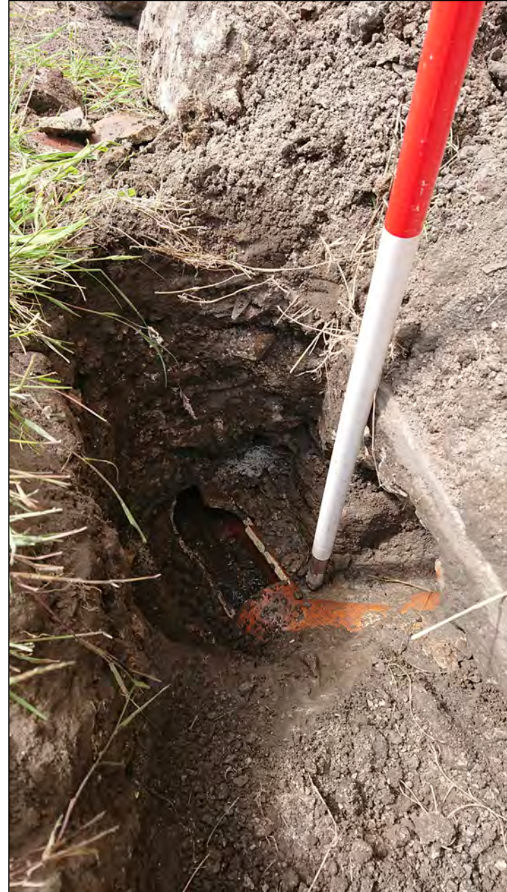
Photo 12. Detail of existing ceramic drain in GY07.
