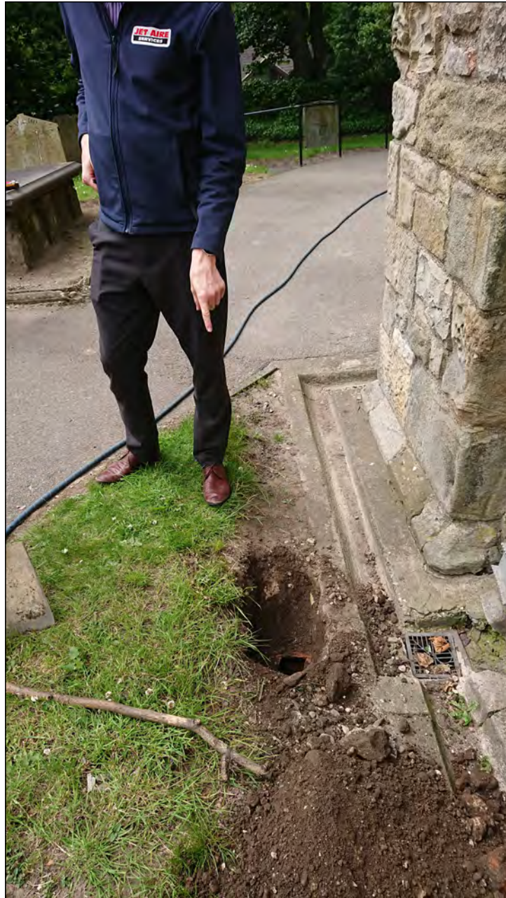
Photo 13. View looking west at Drainage excavation GY08.
