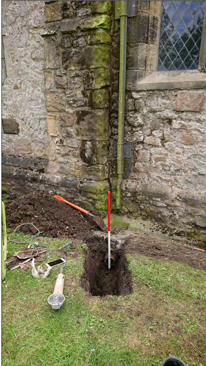
Photo 03. Broad view looking southeast towards Drainage excavation GY02.
