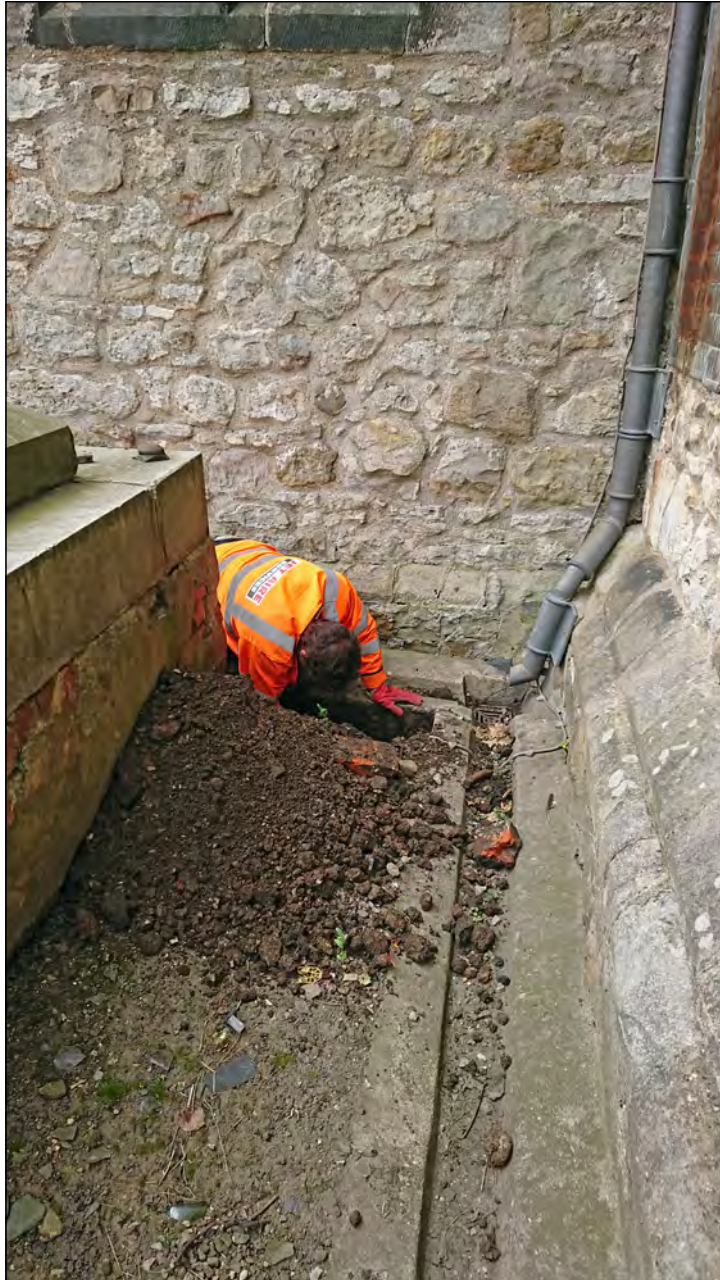
Photo 07. Broad view looking west towards Drainage excavation GY06.
