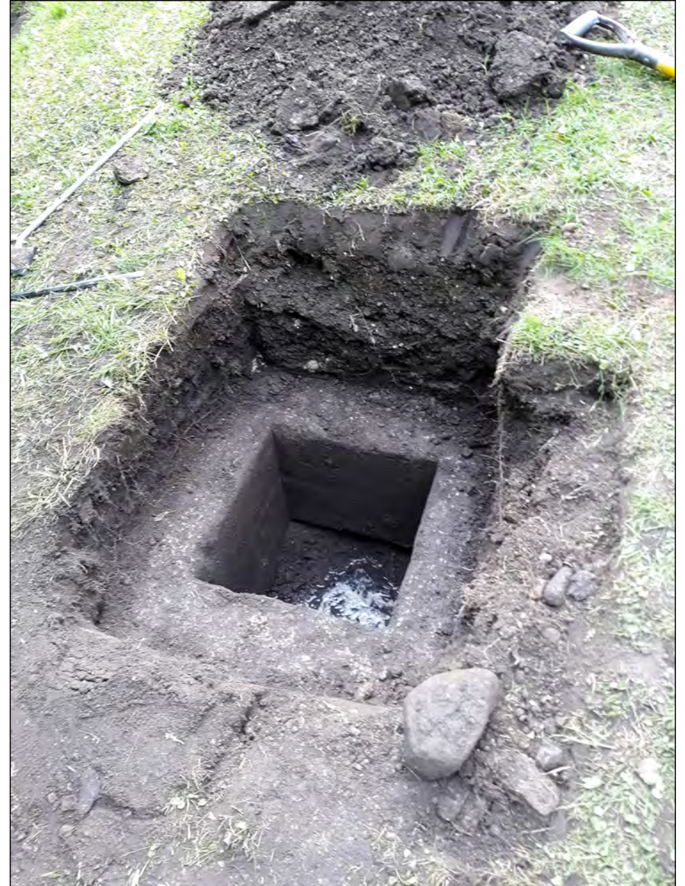
Photo 19. View looking ENE at second (successful) excavation attempt to find MH1.
