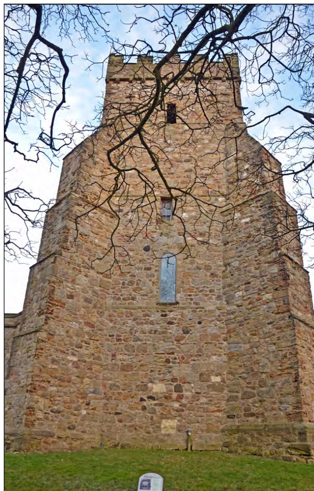
The tower with its massive corner buttresses
