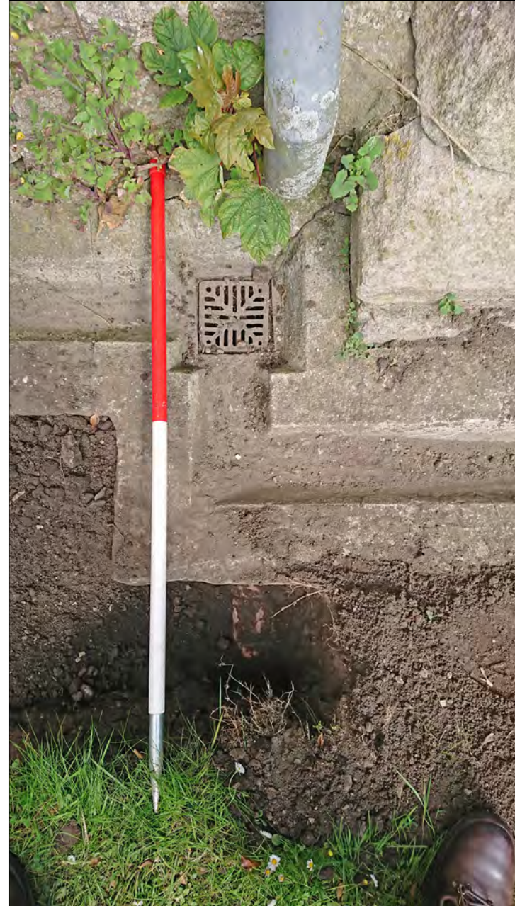
Photo 06. View looking north at Drainage excavation GY05.
