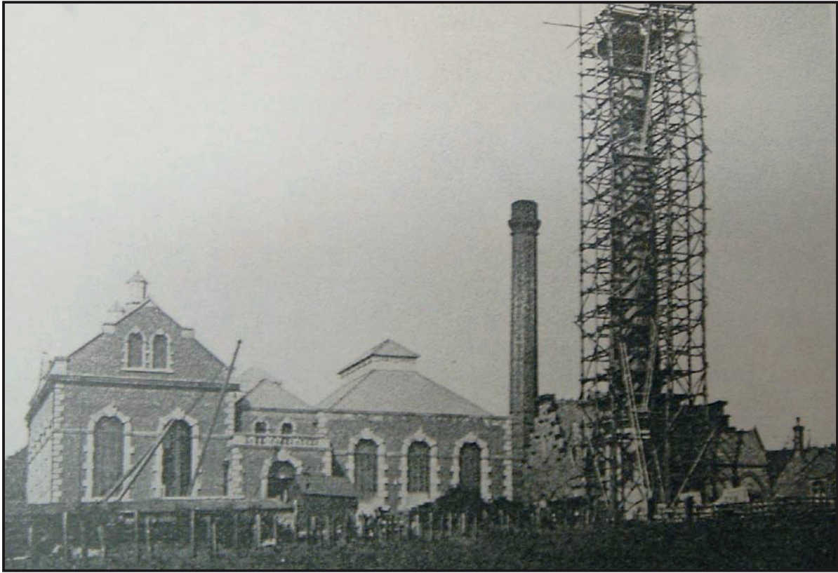
Illus. 17: The construction of Benwell pumping station c.1902. The older building and chimney is shown to the right of the photograph (Rennison 1979, fig 38).
