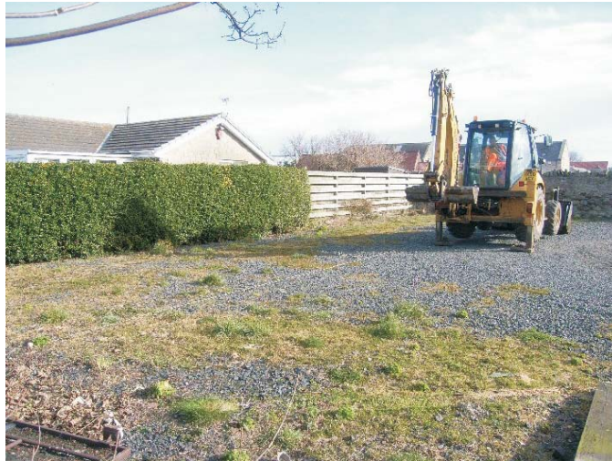
Illus. 09: The position of Trench 1 prior to excavation.
