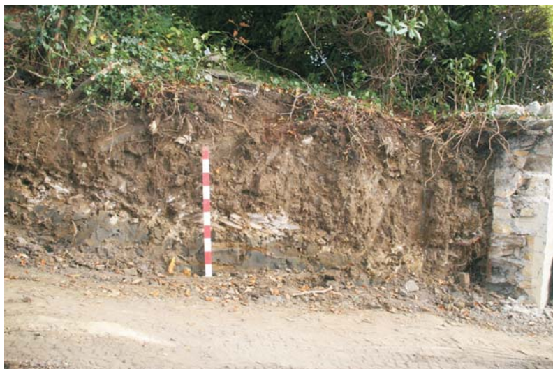
Illus. 12: Detailed view of the west side of the access road (above) into Ingleboro from St Helen's Lane, October 2007.
