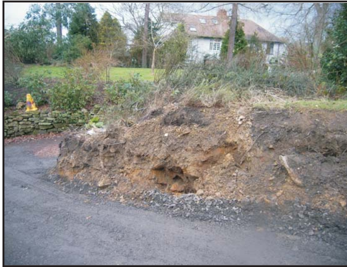
Illus. 13: View south-west from the new property access road adjacent to the new garage towards the original access road (bordered by drystone wall) showing topsoil and sandy subsoil.
