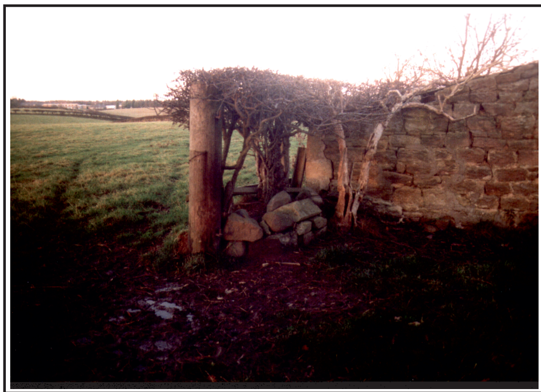
Plate 11: Enclosure fence at East Lane End, showing stone wall of earlier phase of the boundary
