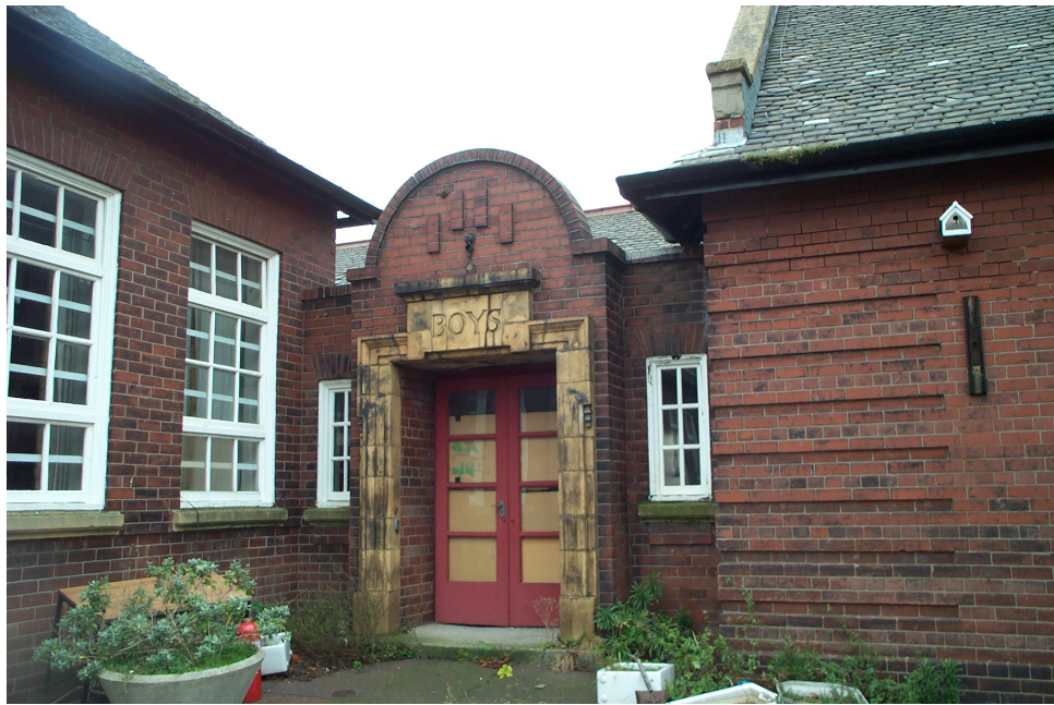
Frontispiece: Moulded brick doorway and surrounding ornamental brickwork in the Central School courtyard
