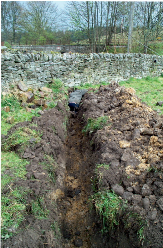
Plate 4: Excavation of ancillary service trench south of the construction site
