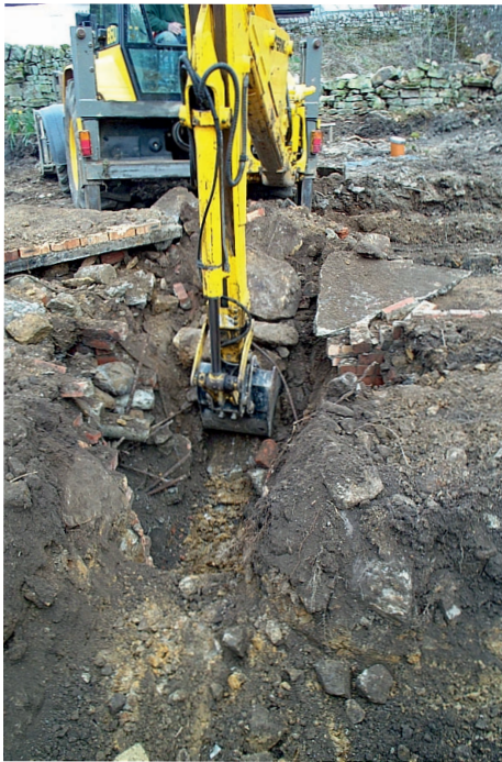
Plate 1: Remains of the old garage, Falstone
