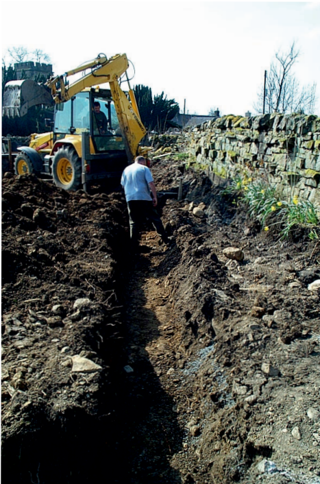
Plate 2: Excavating foundation trench along north wall of the Old Garage site
