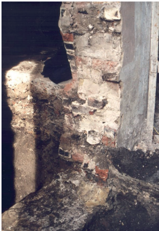
Plate 3: View from E of stone foundation directly underlying brick wall
