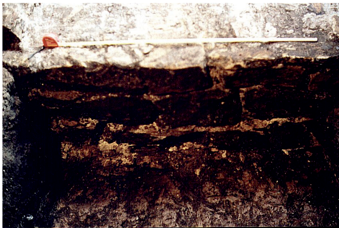
Plate 5: Close-up view of stone foundation wall from the north
