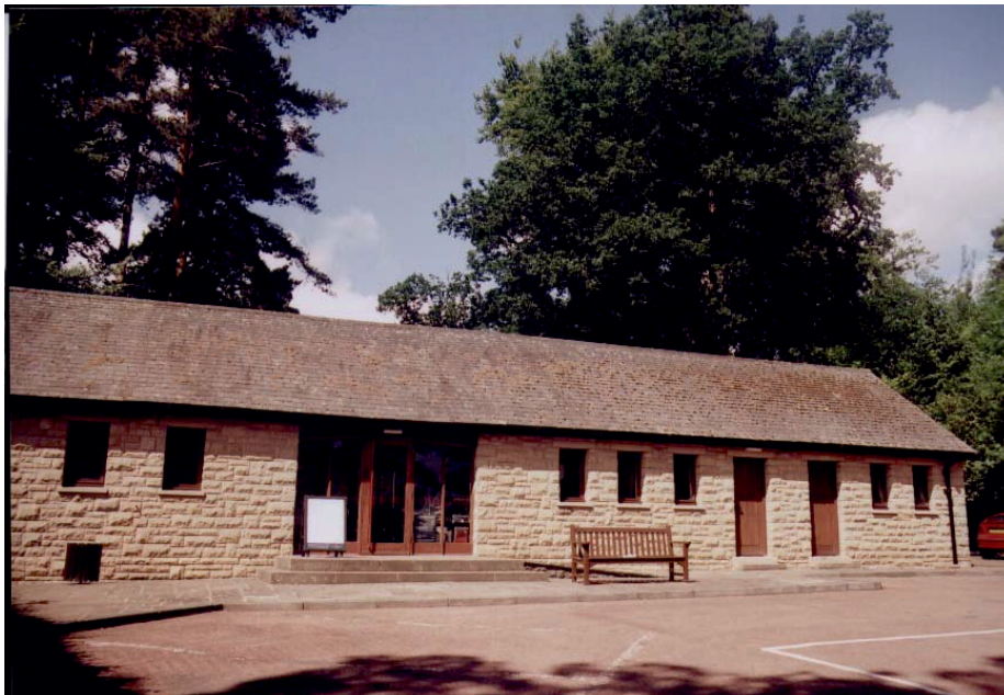
Plate 2: The ticket office/shop from the east
