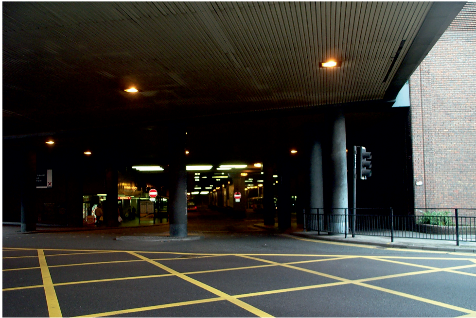
Plate 2: View from Percy Street into the bus concourse, showing sloping levels
