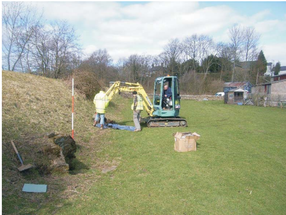
Illus. 16: The position of Trench 3 prior to excavation, viewed from the south-east.
