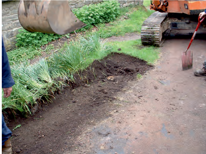
Plate 2: Soil removal for the creation of a footpath.
