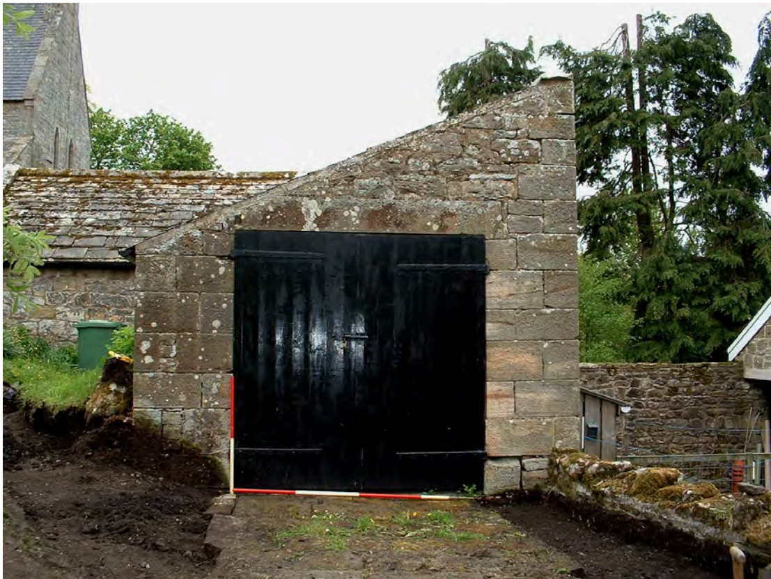
Frontispiece: The vicarage garage doors, showing removal of built-up soil from the wall
