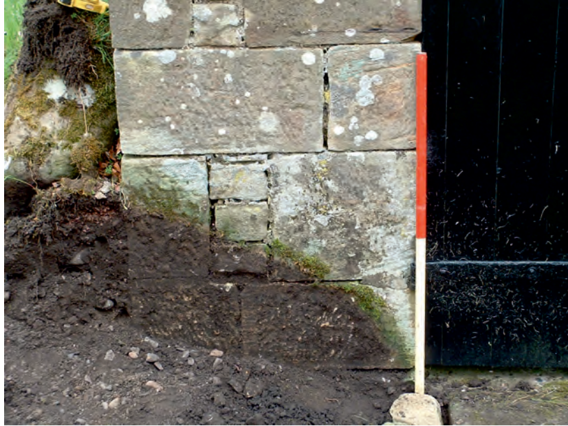
Plate 4: Soil removal for the creation of a footpath, showing the build-up of soil removed from the vicarage garage wall.
