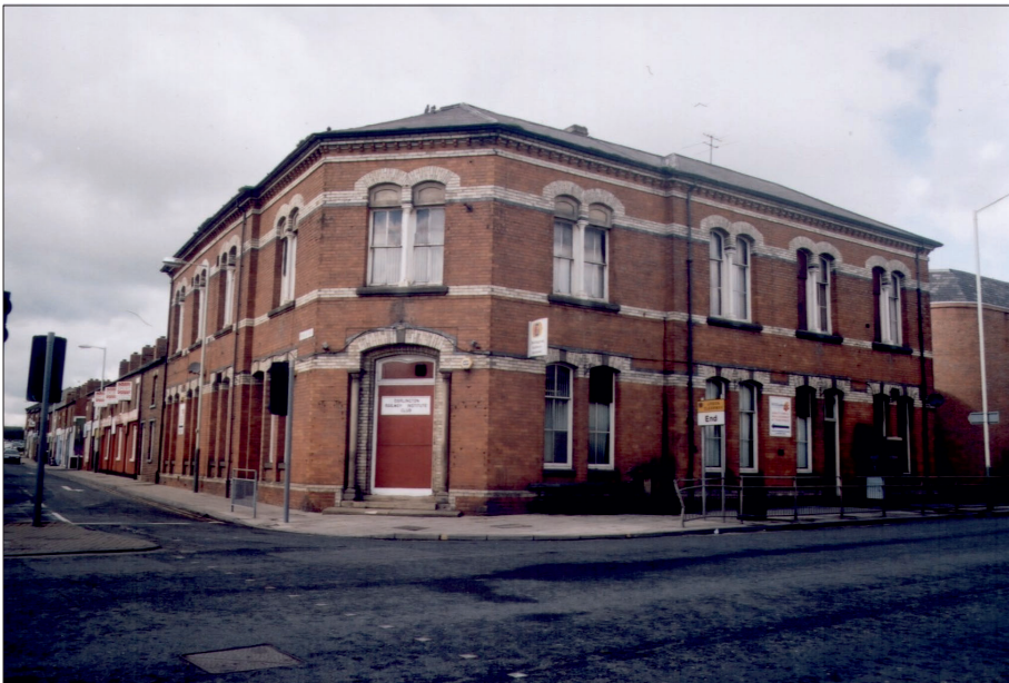
Illustration 20: The Railway Institute building on the corner of Whessoe Road and North Road
