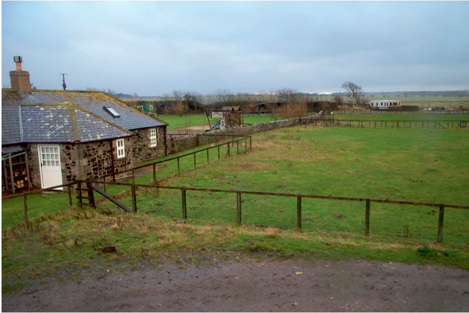
Plate 7: View of the southern boundary of the assessment site from the east
