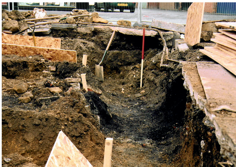
Plate 2: View from South towards the North-East corner of the site, showing coal dust from former coal bunker
