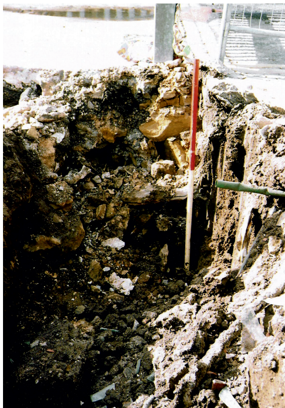
Plate 1: North-West corner of site, viewed from the east - note remains of wall (in section) on roadside.
