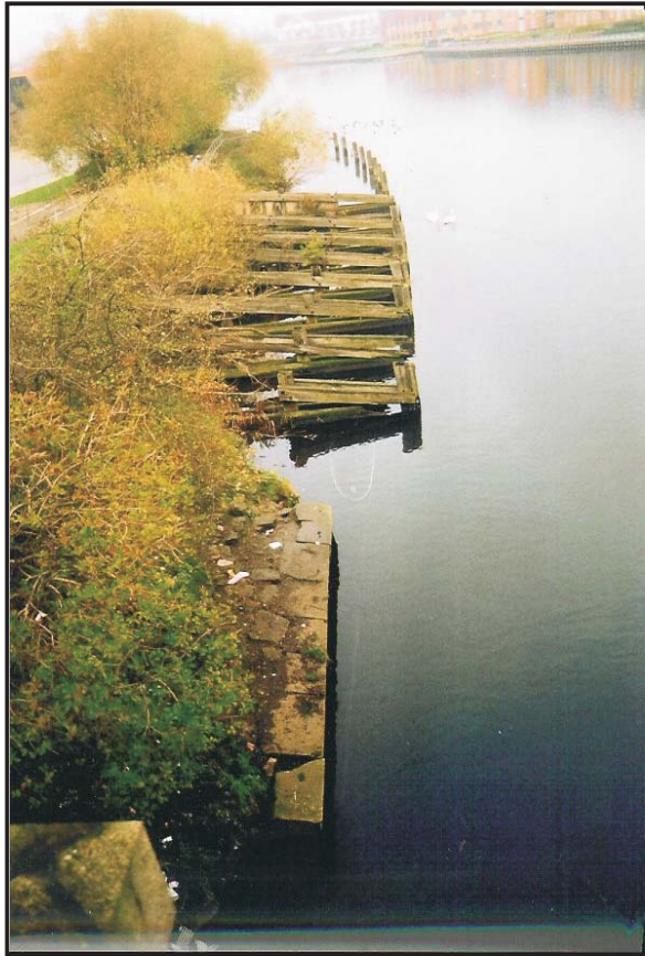
Illus 21: The west abutment of the 1764 bridge viewed from Victoria Bridge
