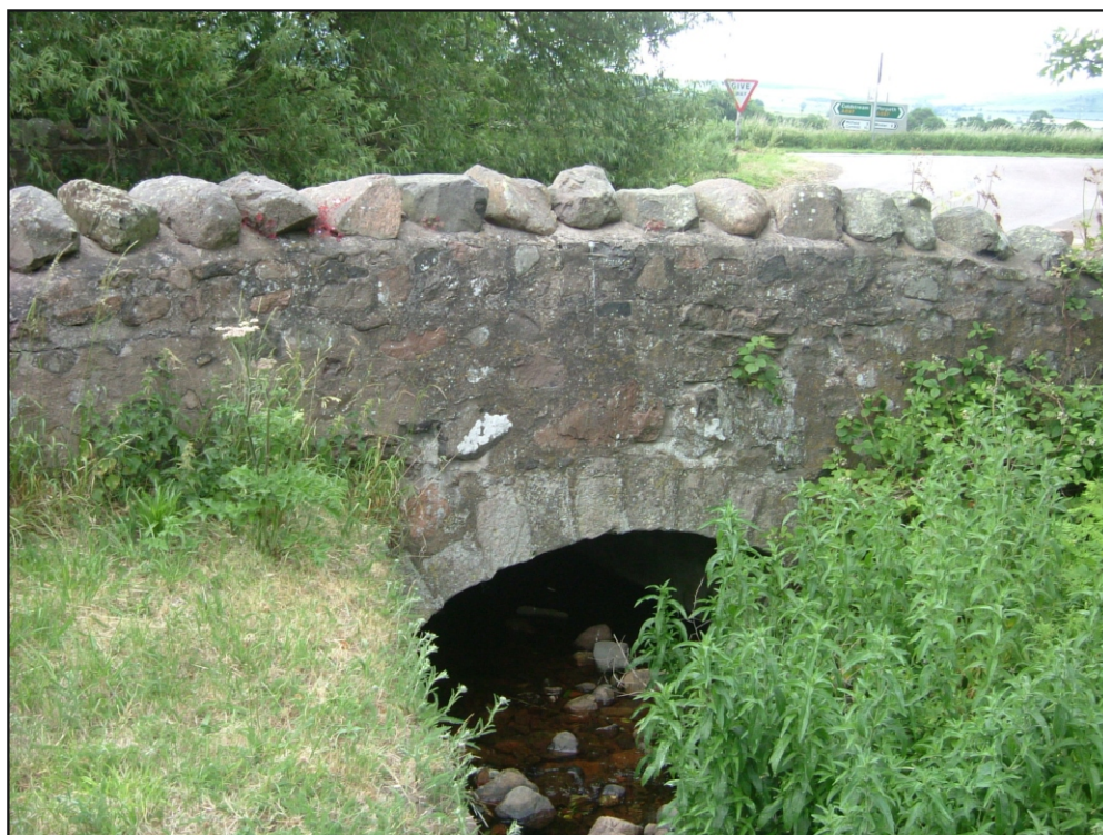
Fig. 30: Akeld Bridge, AK_MP 003
