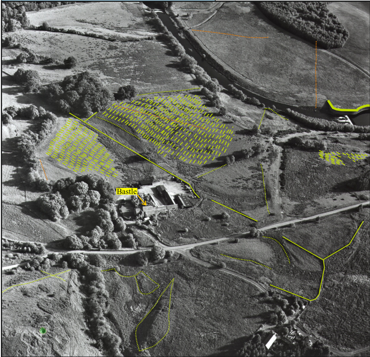
Fig. 11: Aerial view of Hawkehope near Falstone from the north, marking features of potential interest, including the bastle site, ridge & furrow cultivation features close to the farm and walling at the top of Kielder Dam run-off channel.
