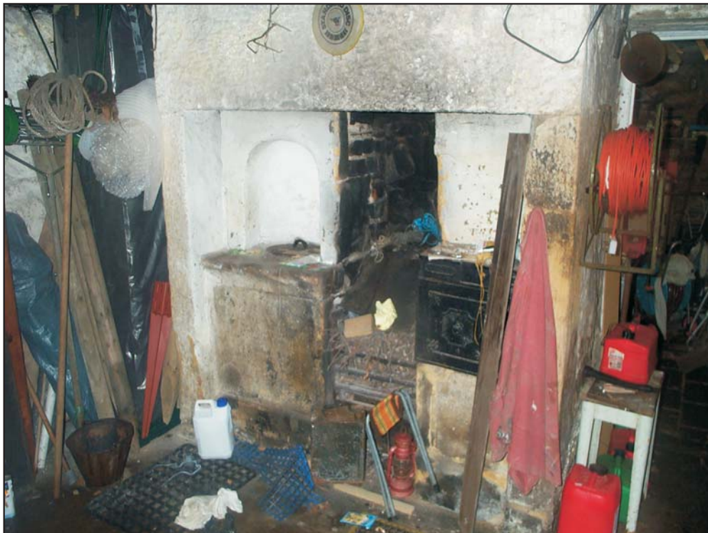
Fig. 55: Fireplace in barn associated with Woodbine Cottage (HOL_MP 104)
