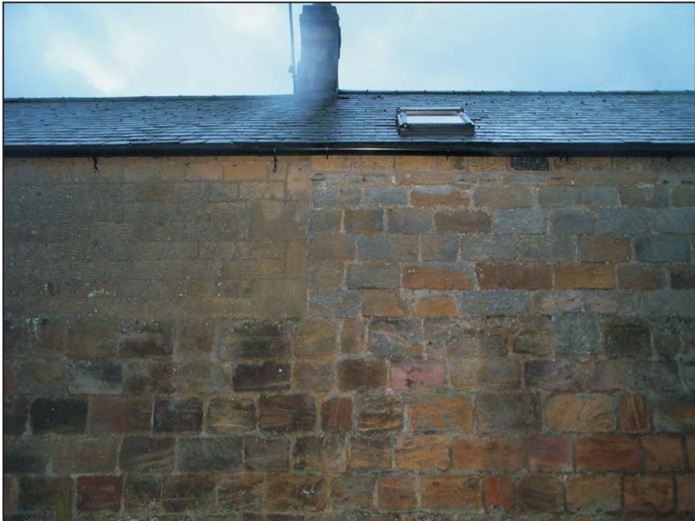
Fig. 51: Holystone mill, detail of masonry (HOL_MP 112)
