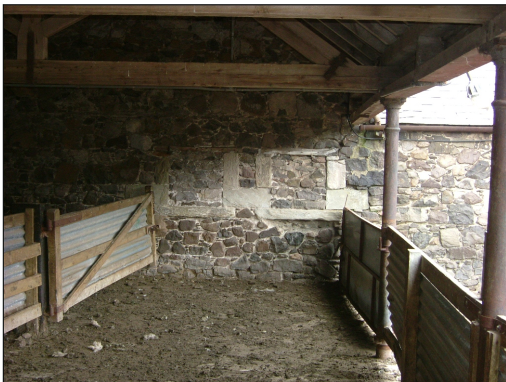
Fig. 48: Blocked windows in farmbuilding, Kilham Farm (KIL_MP 013)
