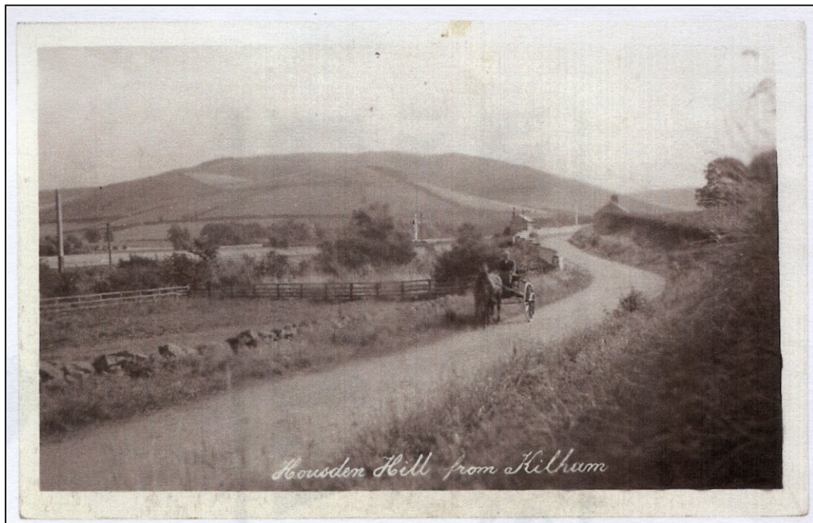
Fig. 45: View of the railway line at Kilham, with a pony & trap on the road and Housden Hill in the background, c.1900 (KIL_HP 004)
