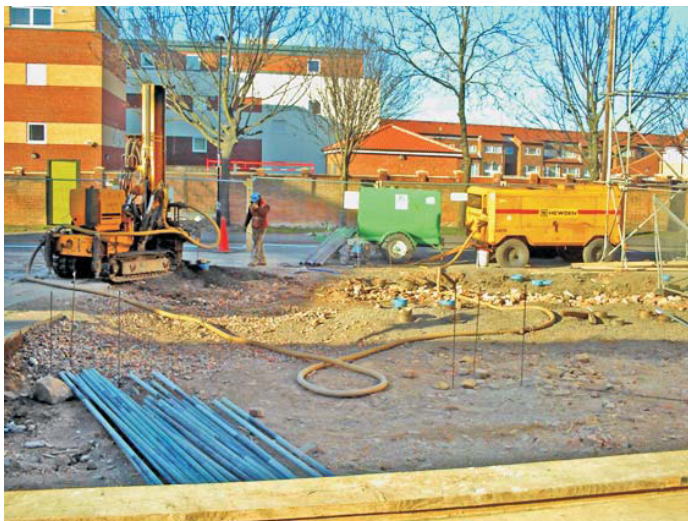
Illus. 08: View of the site from the south.
