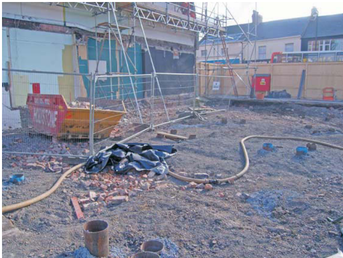
Illus. 10: View across the site towards Shields Road from the north.
