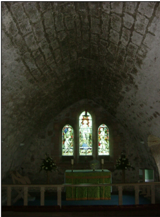
Fig. 66: St Gregory's church, vaulted chancel (KN_MP 025)
