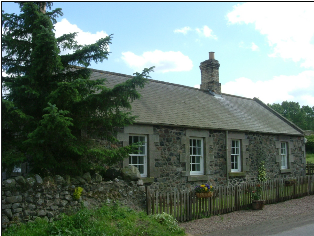
Fig. 85: Cottage, Westnewton (WN_MP 034)
