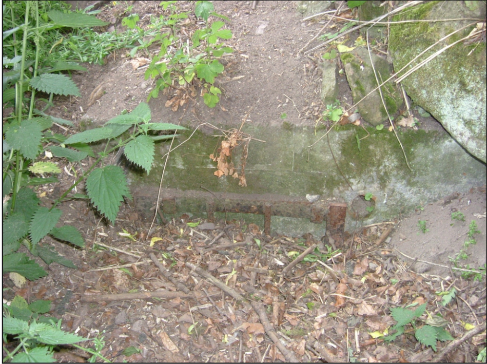
Fig. 72: Remains of sluice (WN_MP 002)
