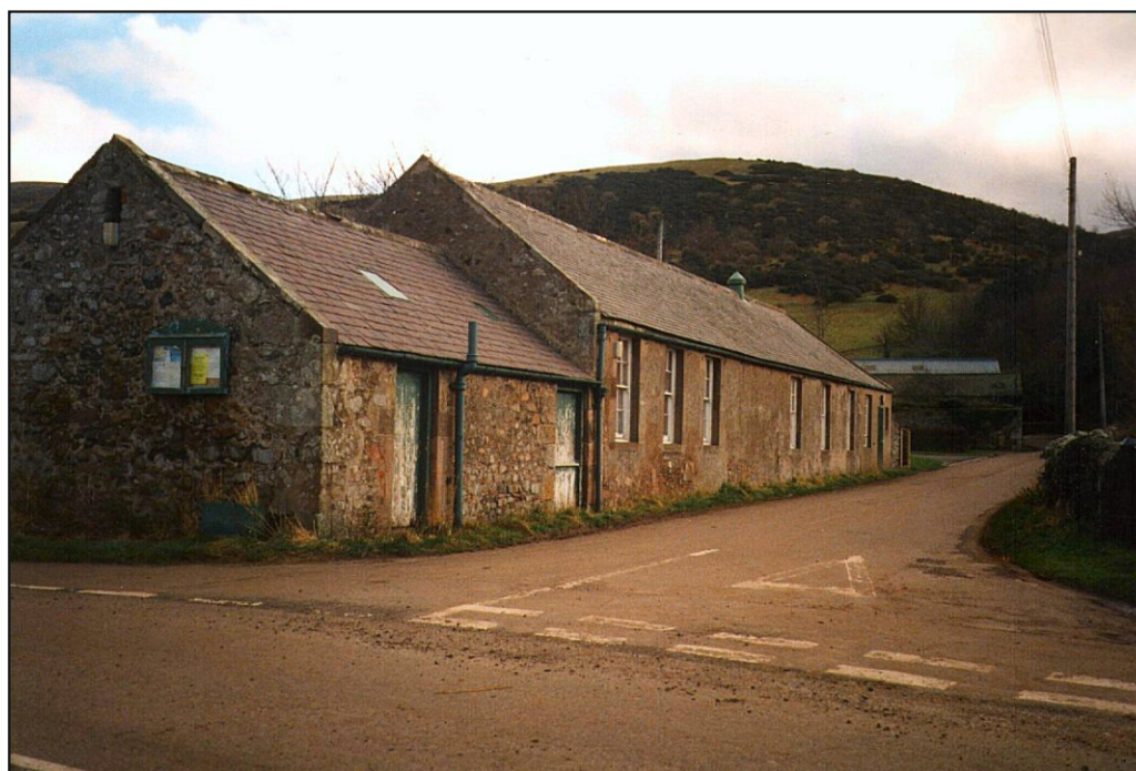
Fig. 58: Kirknewton schoolhouse/hall before demolition in the 1990s (KN_HP 013)
