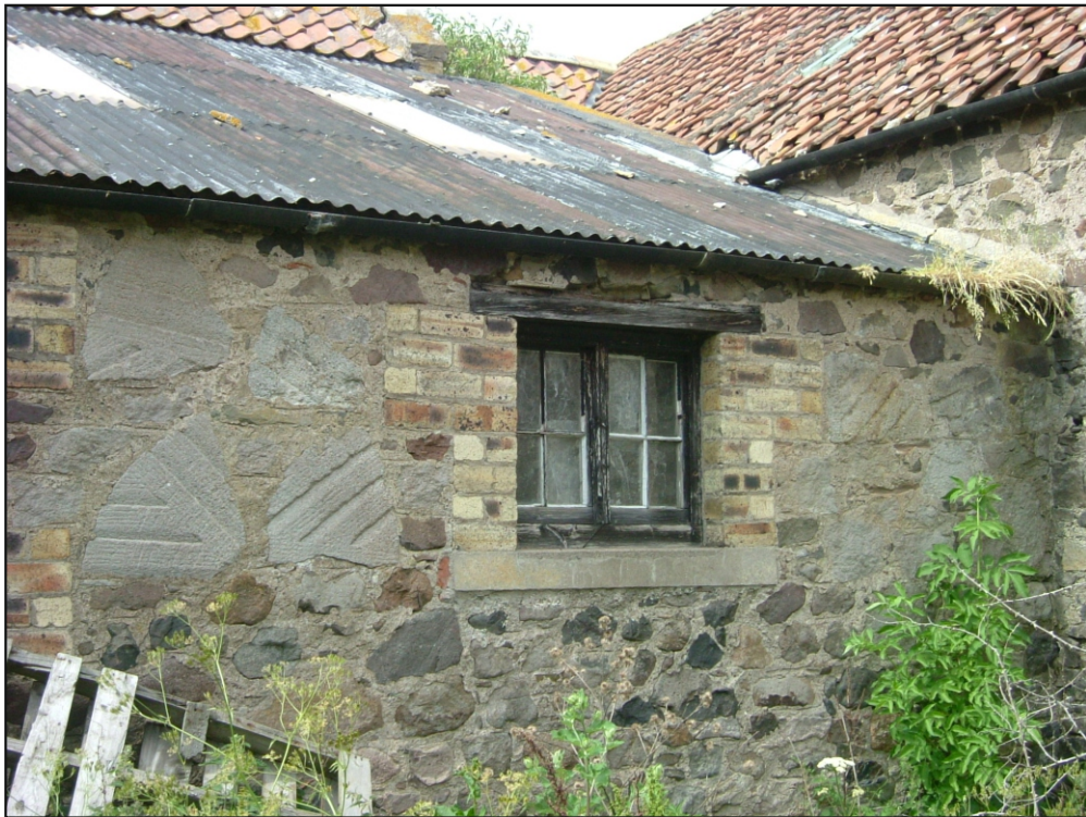
Fig. 73: Millstone fragments reused as masonry (WN_MP 008)
