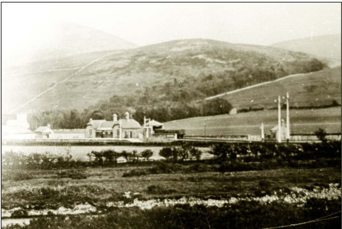
Fig. 56: Distant view of Kirknewton Station, c. 1920 (KN_HP 019)
