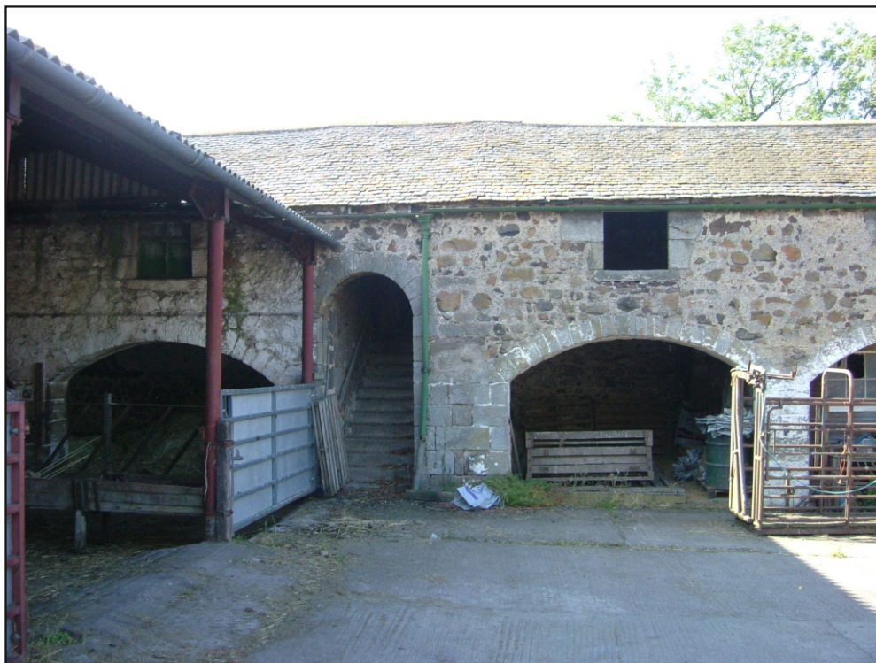
Fig. 67: Farmbuildings at Kirknewton West farm (KN_MP 030)
