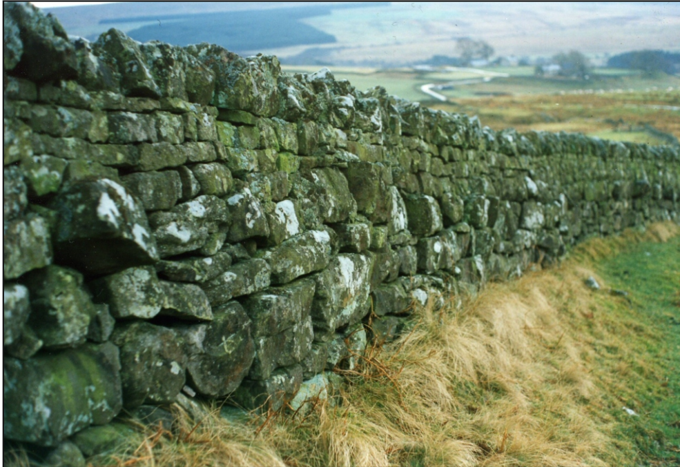
Fig. 71: Multi-phase field wall near Dykehead (RO_MP 107)
