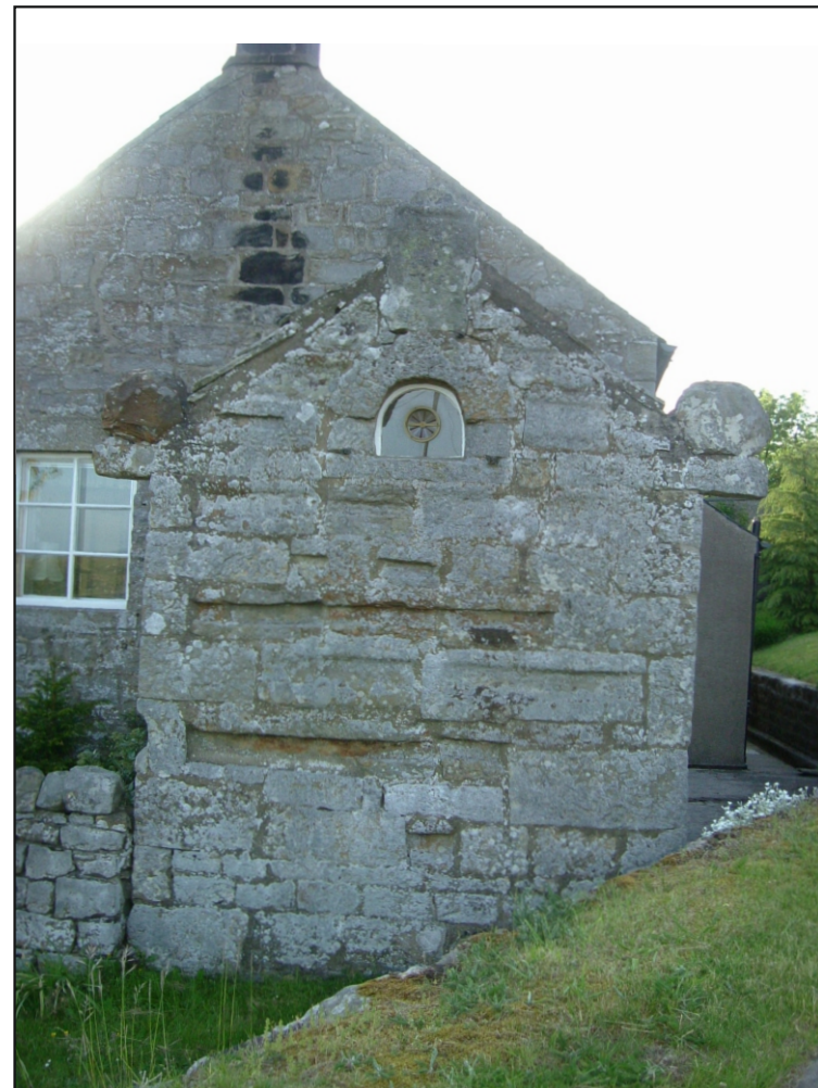
Fig. 66: Roman masonry reused in The Old Schoolhouse (RO_MP 058)
