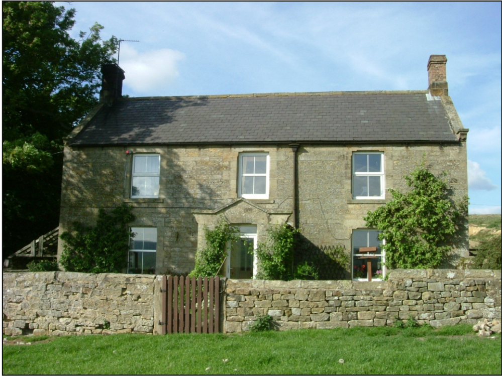
Fig. 57: Dykehead farmhouse (RO_MP 028)
