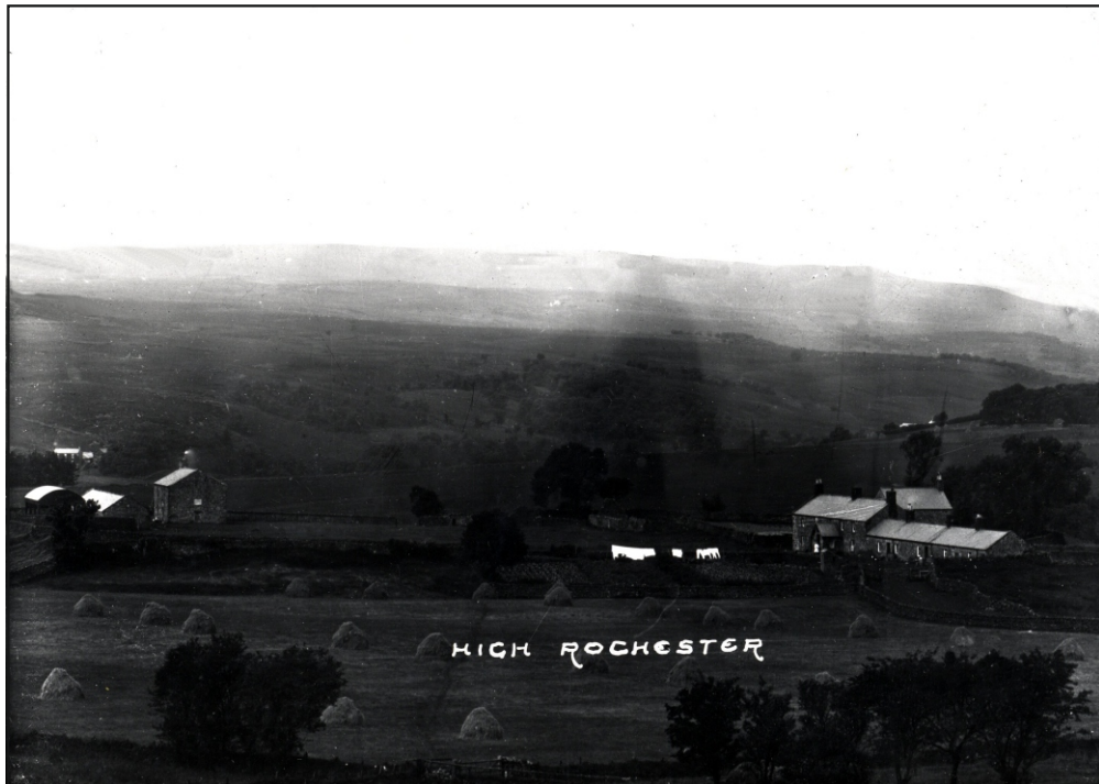
Fig. 49: High Rochester viewed from the East, c.1910 (RO_HP 008)
