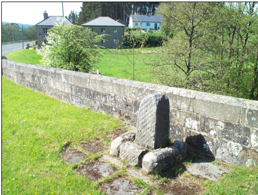
Fig. 67: Milestone on Birdhopecraig bridge (RO_MP 007)
