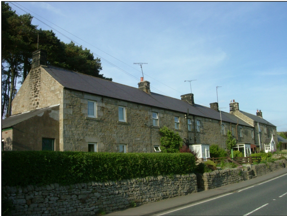
Fig. 60: Redeswater view and attached terrace, Rochester (RO_MP 058)
