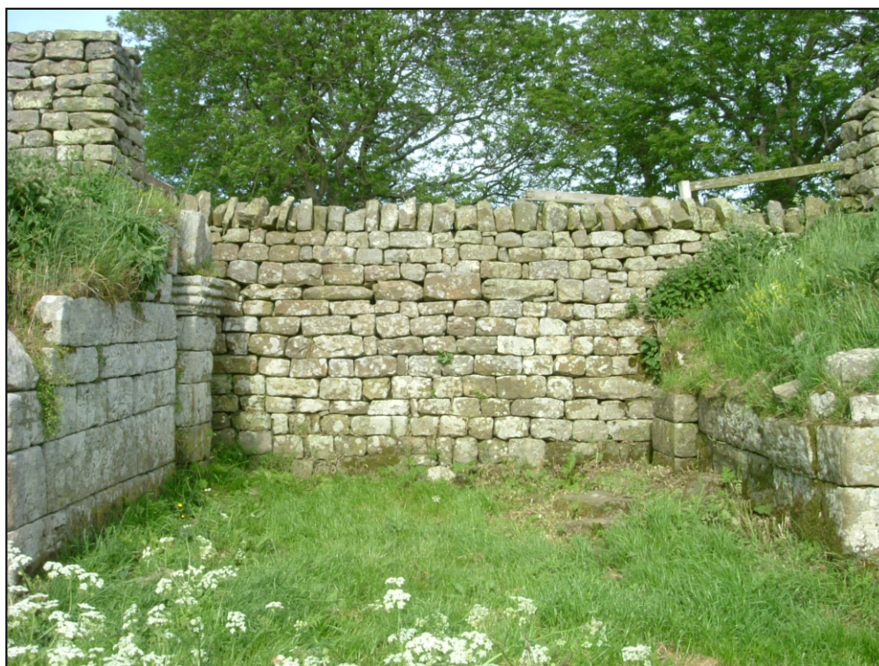
Fig.52: High Rochester Roman Fort, blocked West gate (RO_MP 019)
