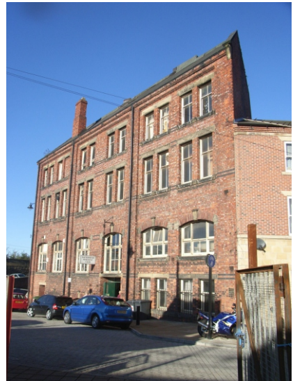
Illus. 09: Gateshead Railway Club, south elevation.
