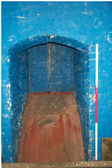
Illus. 16: Cellar coal chute
