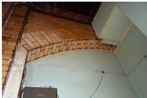
Illus. 19: Original glazed brickwork at first floor level
