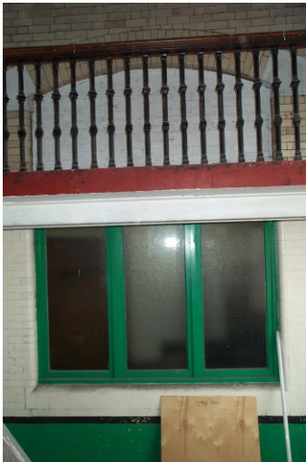
Illus. 26: Top of north-east stair well with walls clad in cream coloured glazed brick
