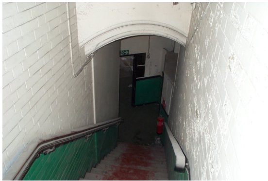
Illus. 22: Back stairs from first to basement (former gymnasium)
