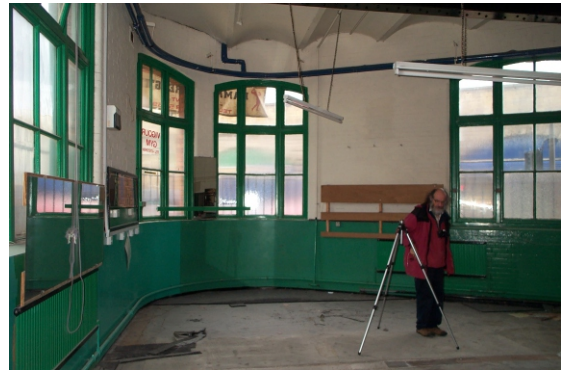
Illus. 21: NW corner of basement (former gymnasium)
