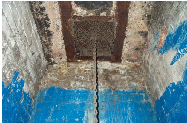
Illus. 17: Entrance to cellar coal chute from street level
