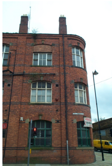
Illus. 11: Gateshead Railway Club, west end of north elevation.
