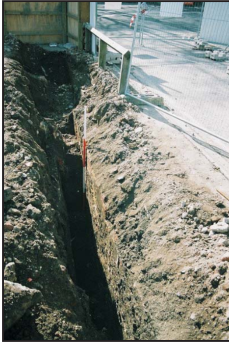
4. Construction trench beside Strawberry Lane looking S towards Gallowgate
