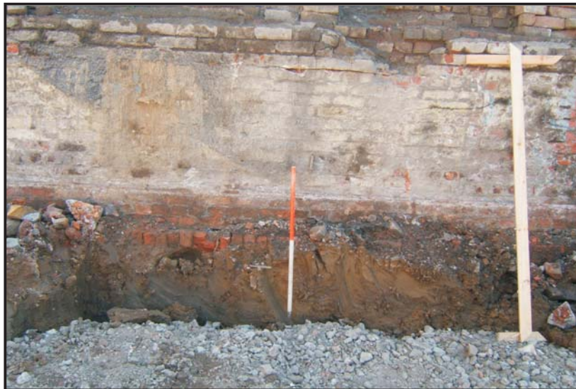
2. Section at the front of the western part of the site (the wall is the front wall of the cellaring for 30-34 Gallowgate)
