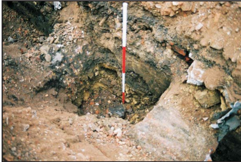
8. Slot between the two brick walls in the piling trench showing the courses of stone walling at the bottom (looking N)
