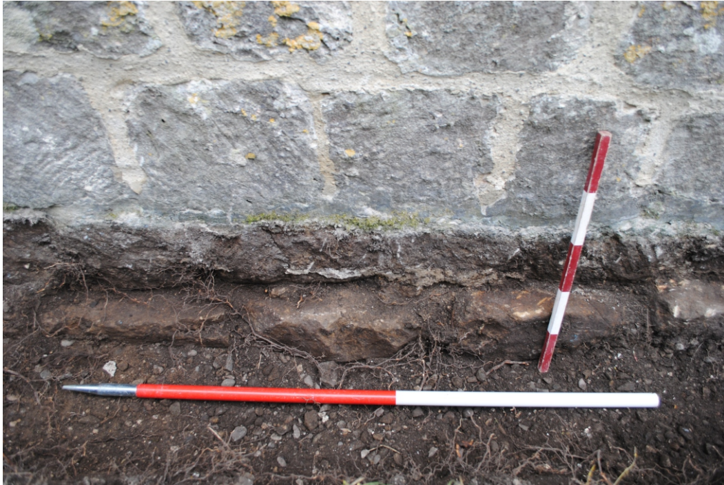
Photo 04. The chancel plinth revealed in excavations for the drain. South view.
