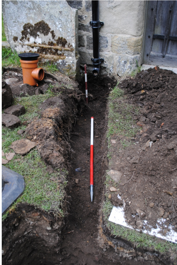
Photo 10. The channel leading from guttering by the church door to soakaway pit 2, looking north-west.
