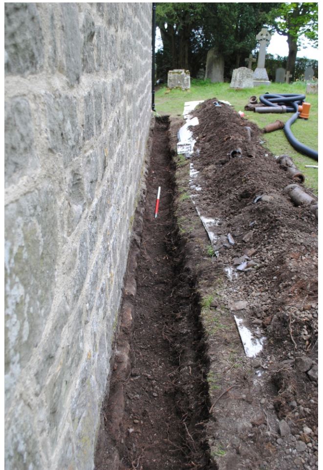
Photo 03. View looking west at excavations for the drain.
