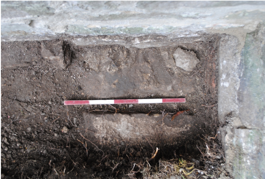
Photo 07. The footing adjacent to the north buttress on the west wall, photographed in plan
