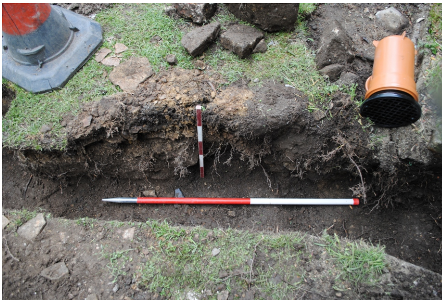
Photo 11. The channel feeding into soakaway pit 2 looking south-west, showing a layer of sandstone rubble.
