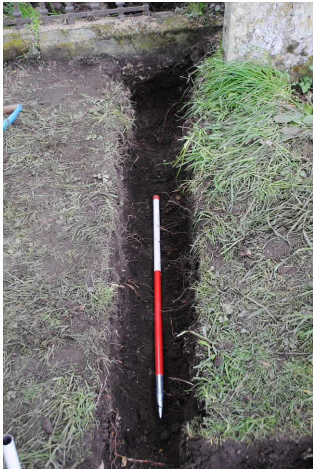
Photo 13. The channel feeding into soakaway pit 3 looking west, showing historical alterations to the memorial plot coping.
